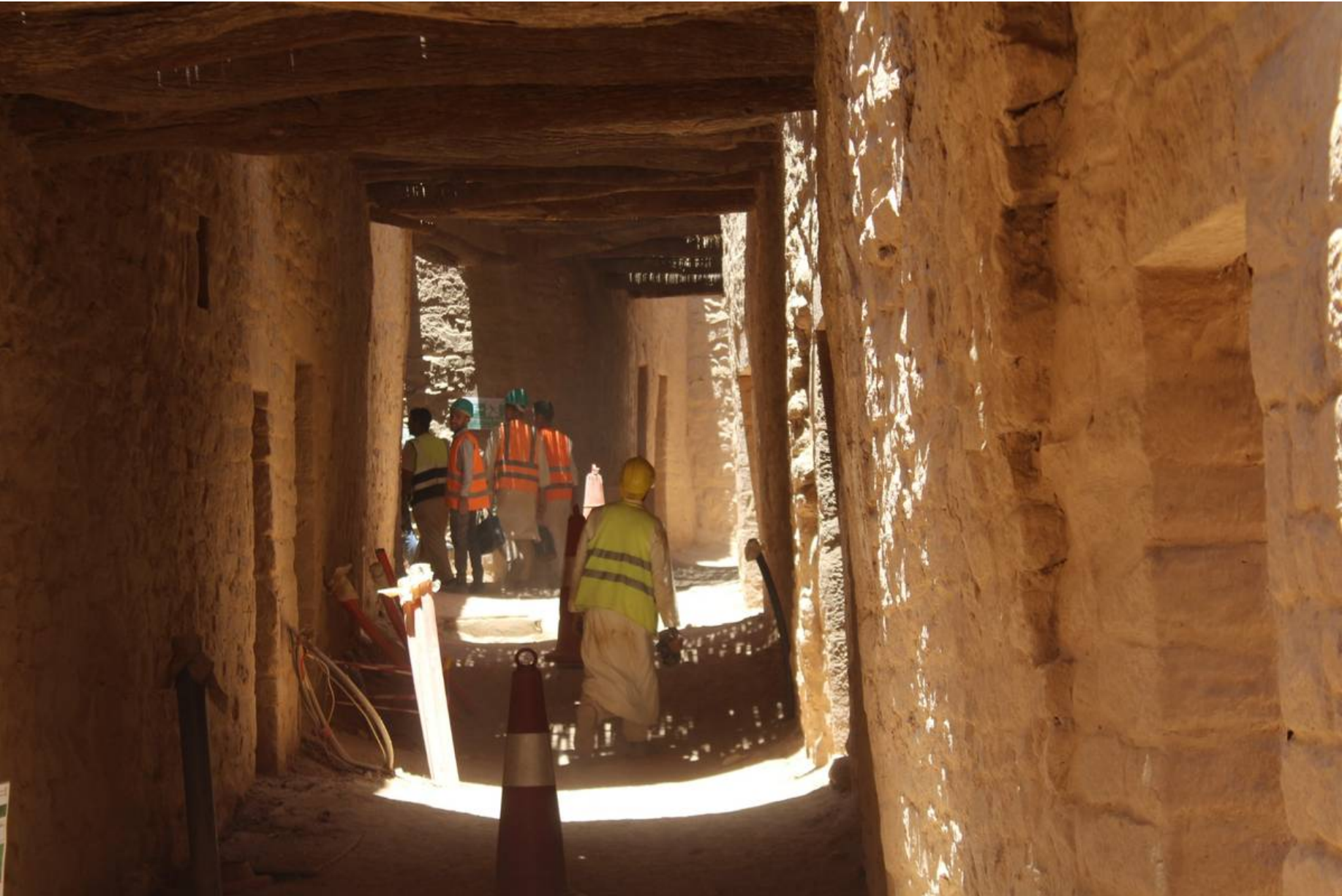
01 Adaptive Reuse Works in Progress
