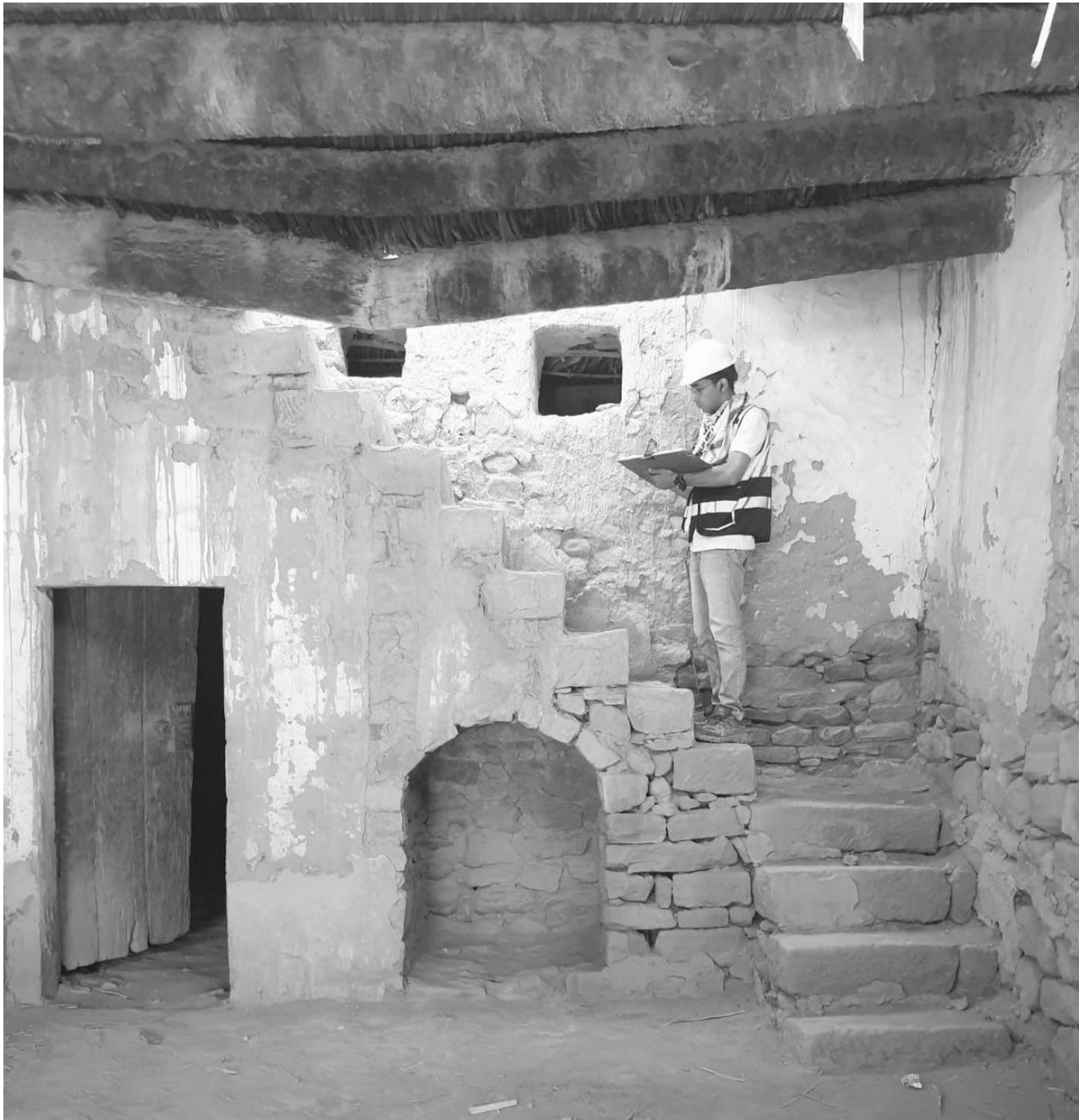
Recording an existing staircase and interior
