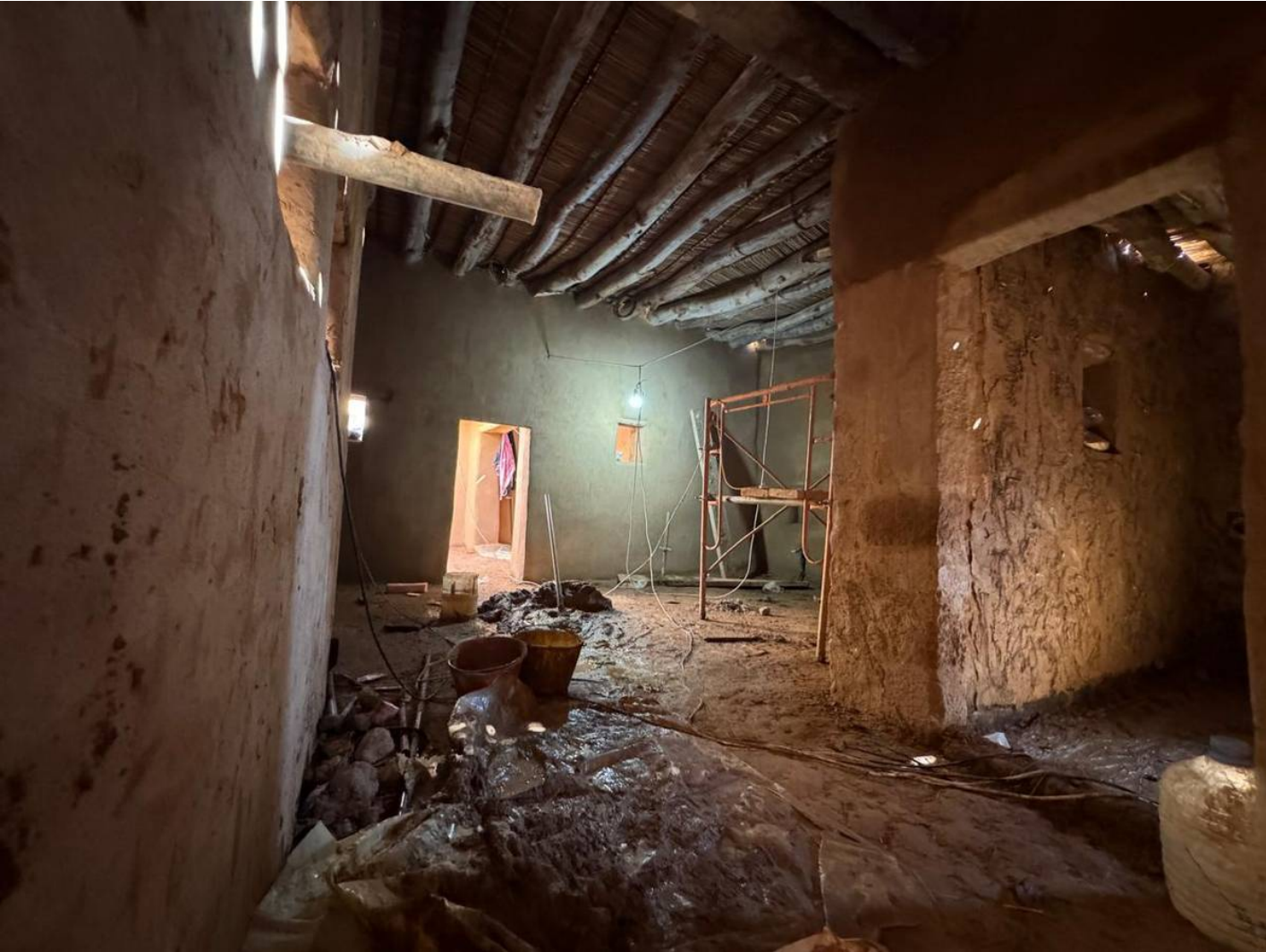
02 Adaptive Reuse Works in Progress
