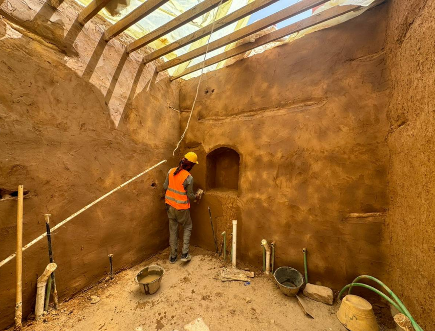
Restoration Works in Progress / View 01
