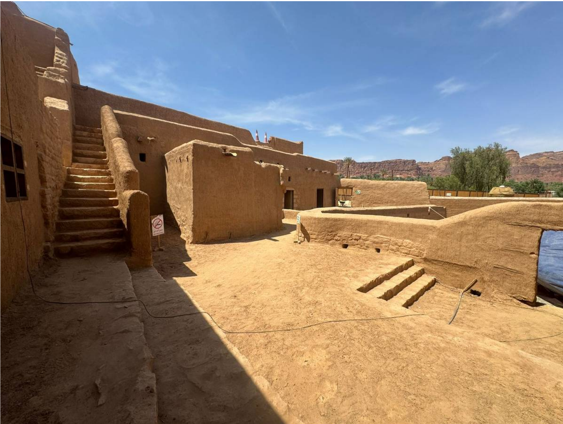
Restored Condition / View 02
