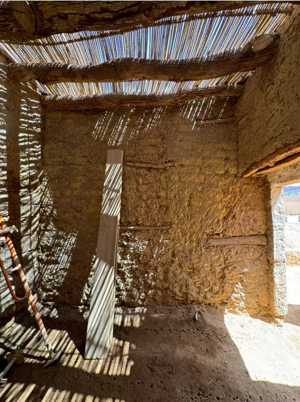
Restoration Works in Progress
