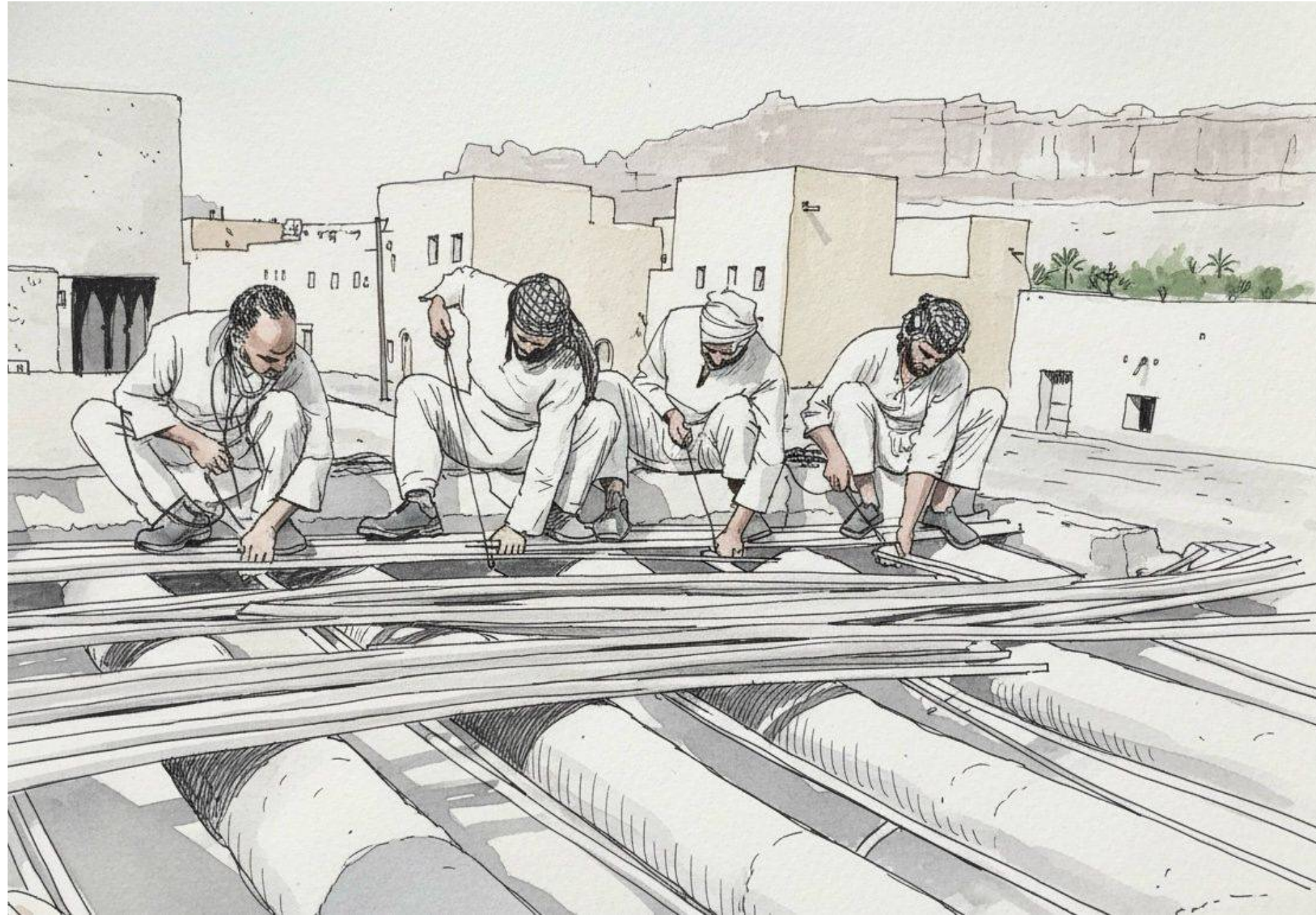
Craftspeople working on a roof
