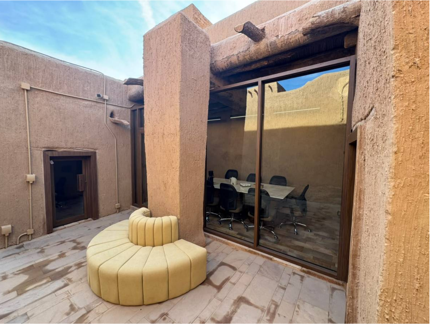
Adaptively Reused Condition
