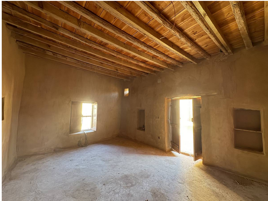
03 Restored Condition - First floor
