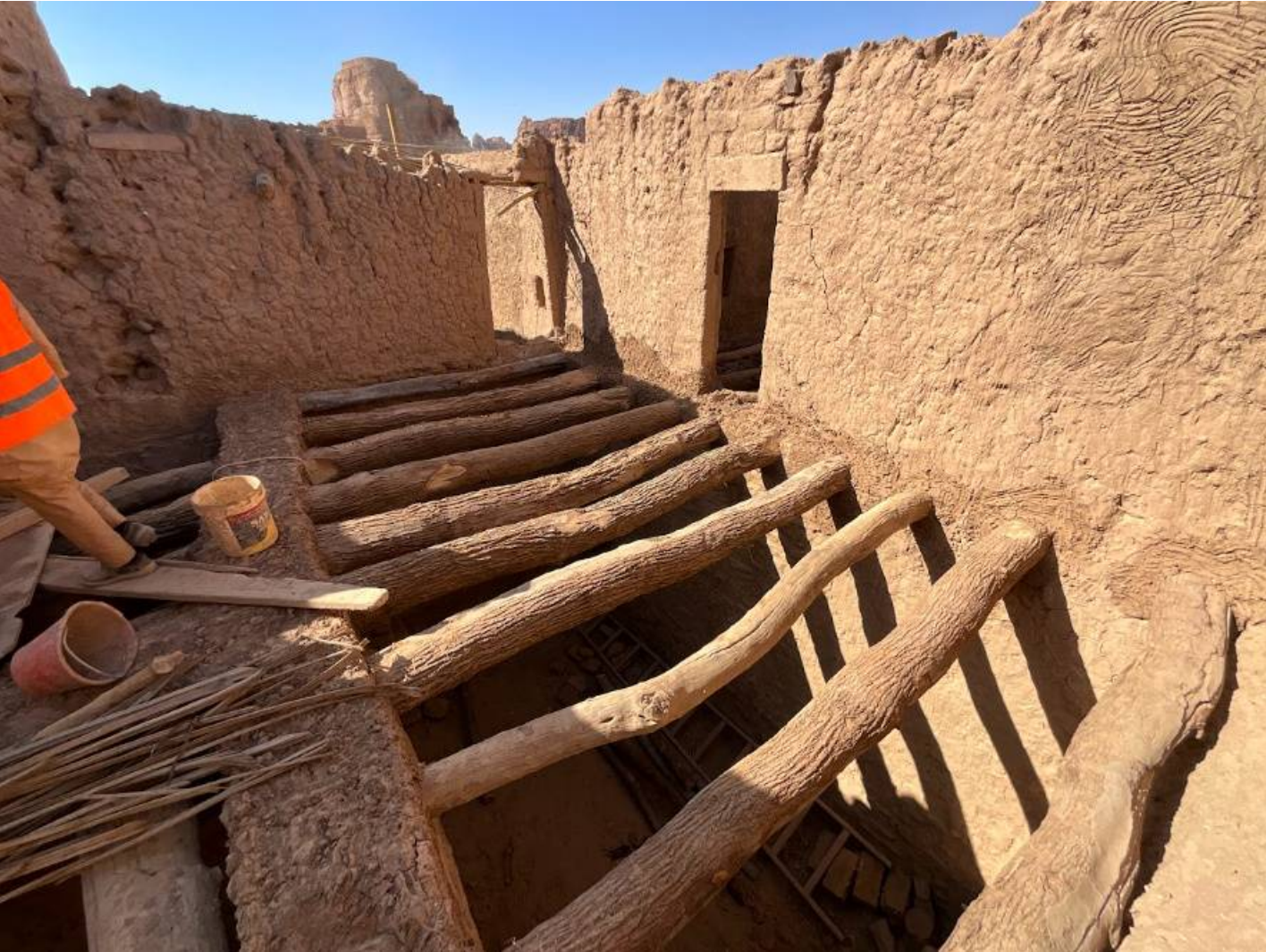
01 Restoration Works in Progress
