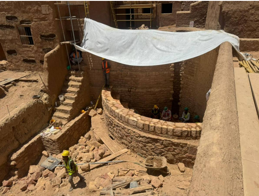
Restoration Works in Progress
