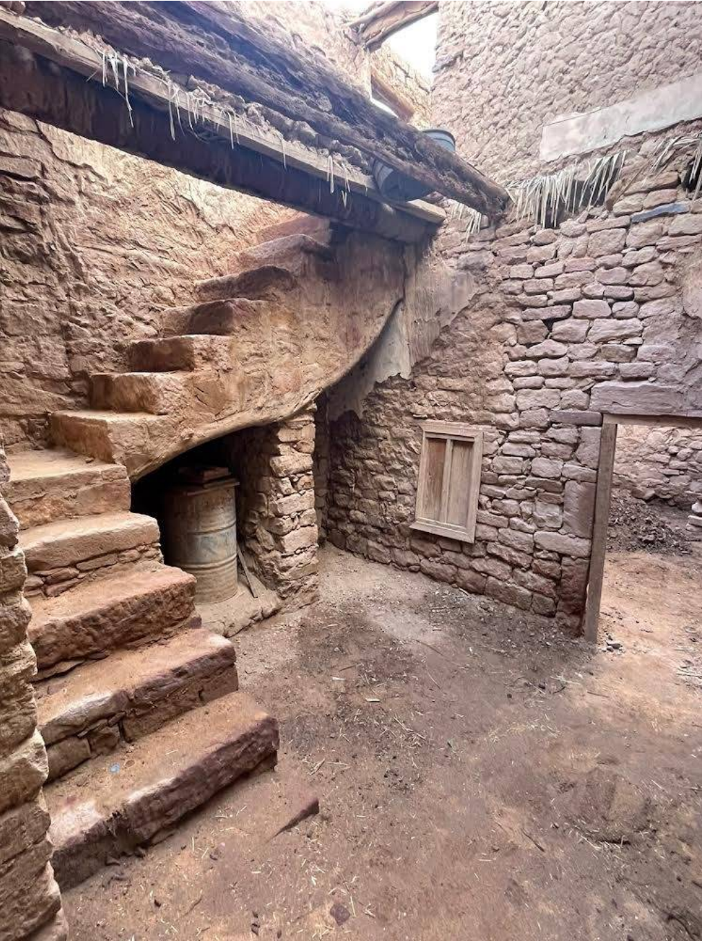
01 Restoration Works in Progress
