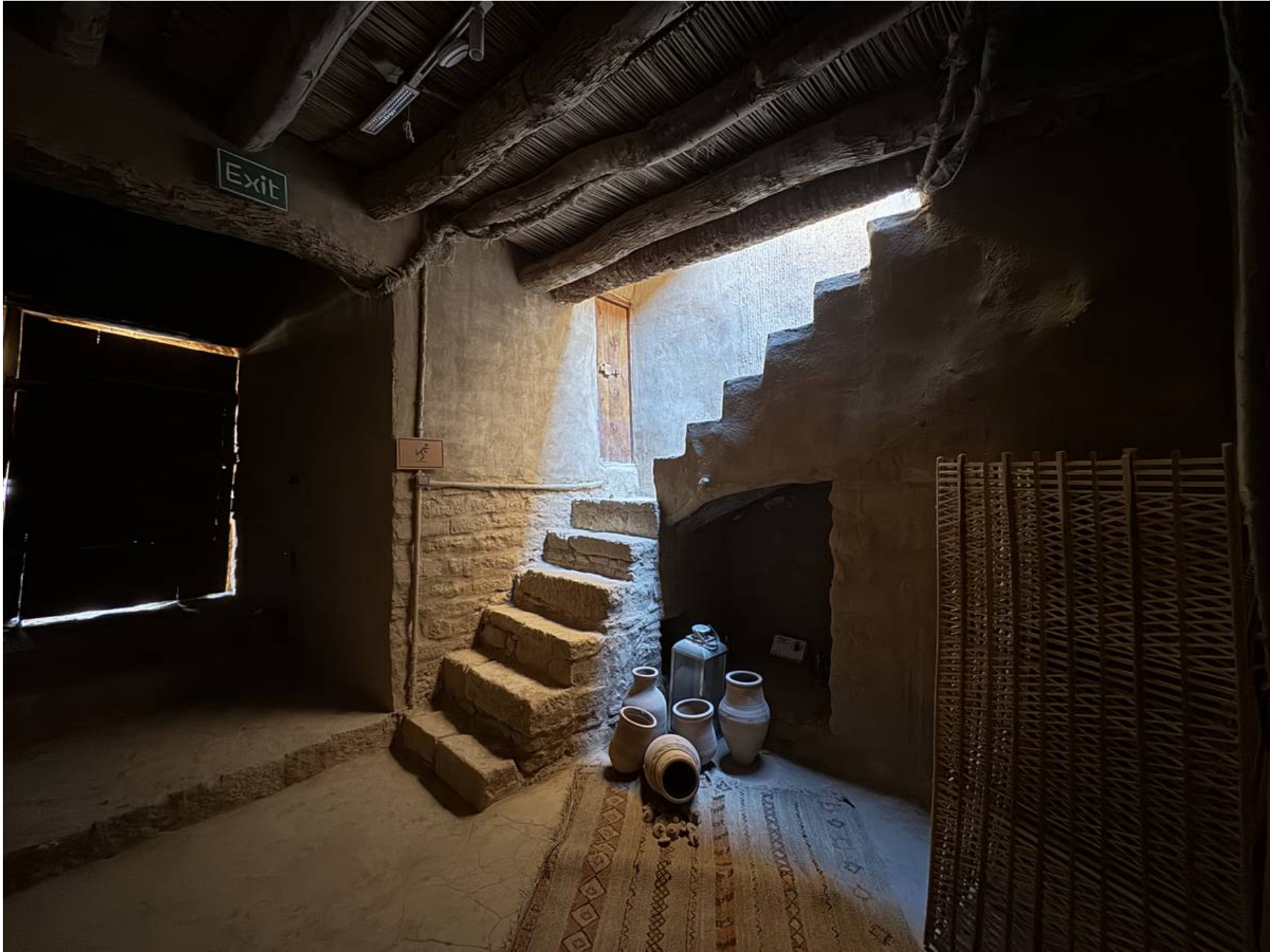
02 Adaptively Reused Condition
