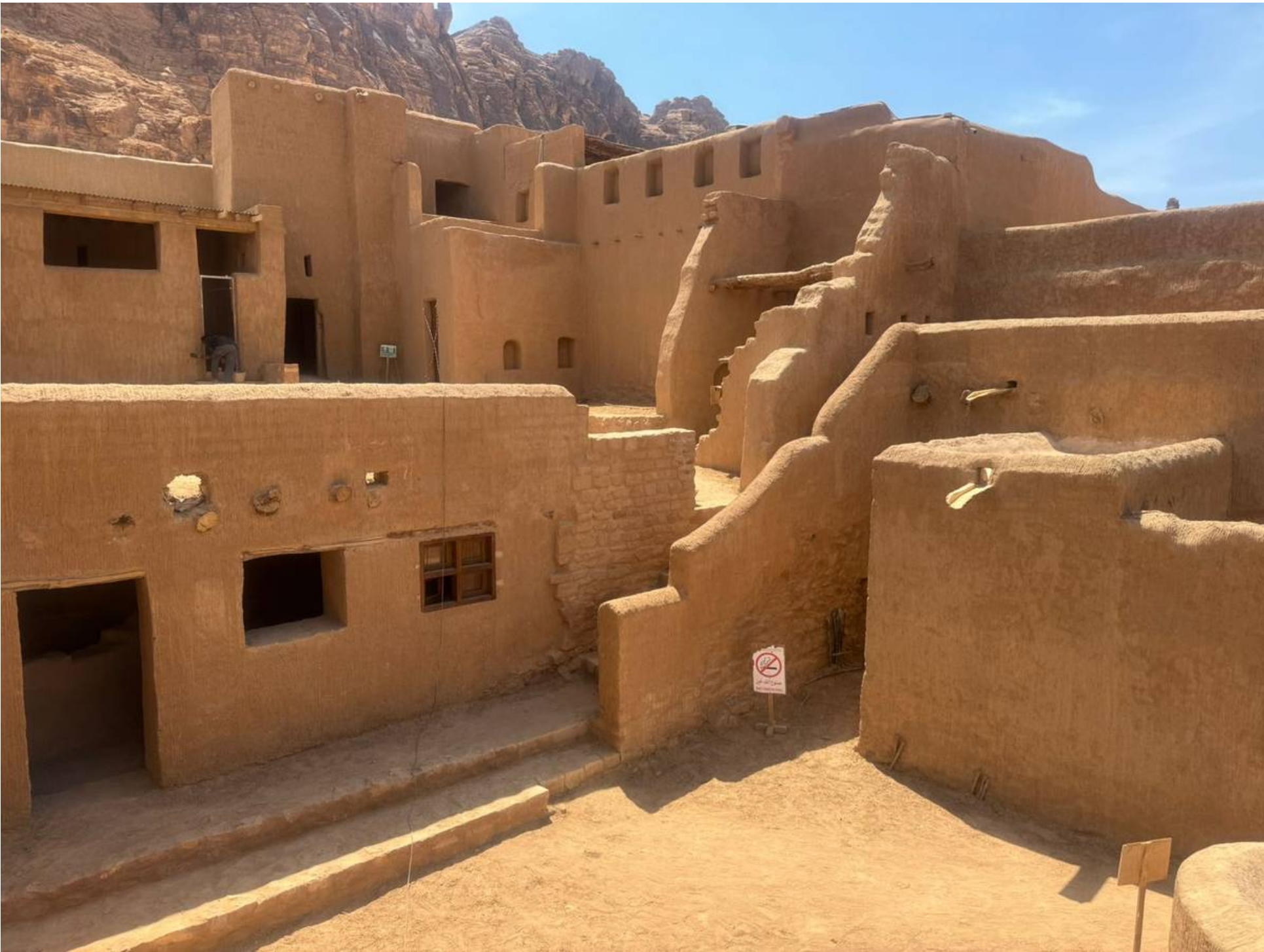
Restored Condition / View 03
