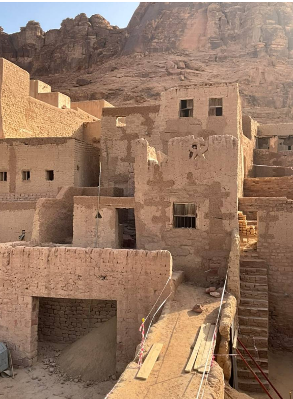
Restoration Works in Progress / View 01
