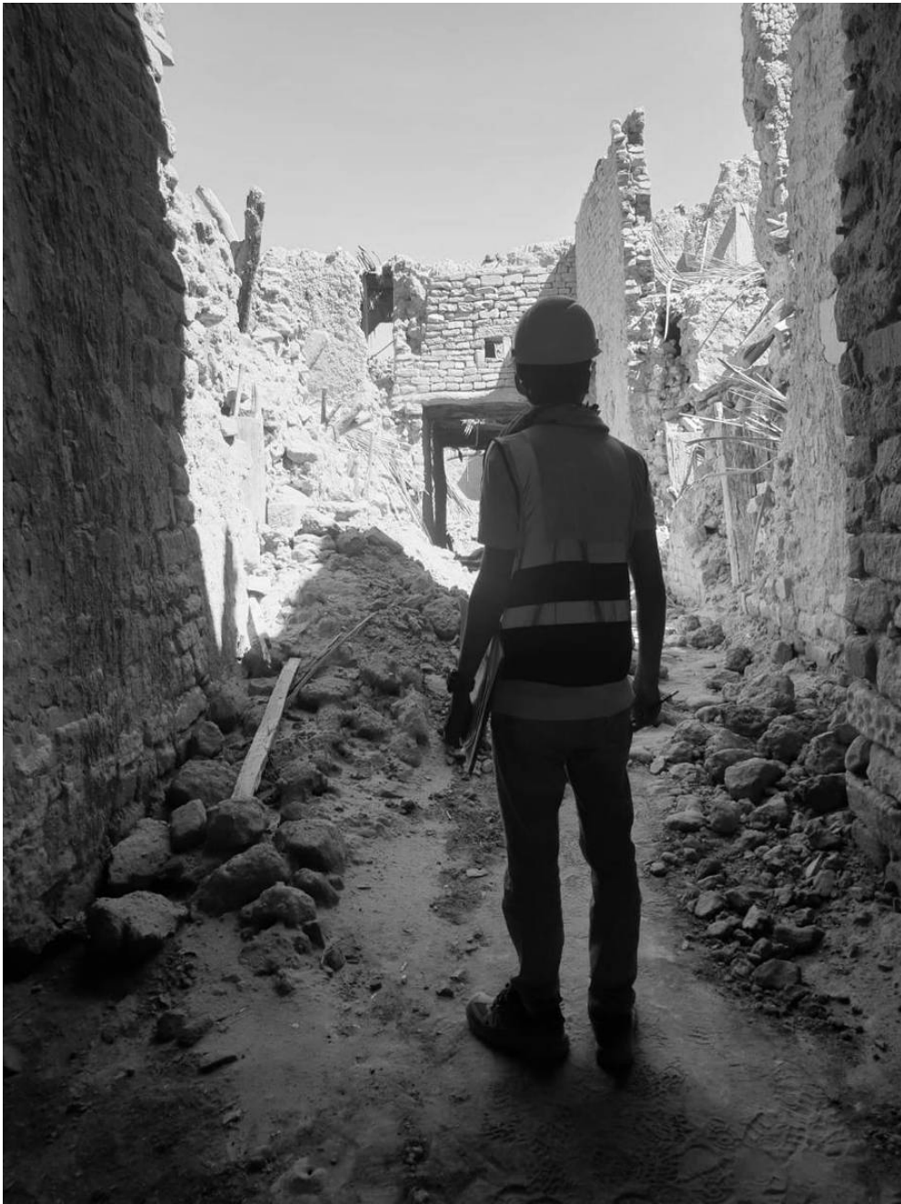
Reviewing existing conditions in the Old Town
