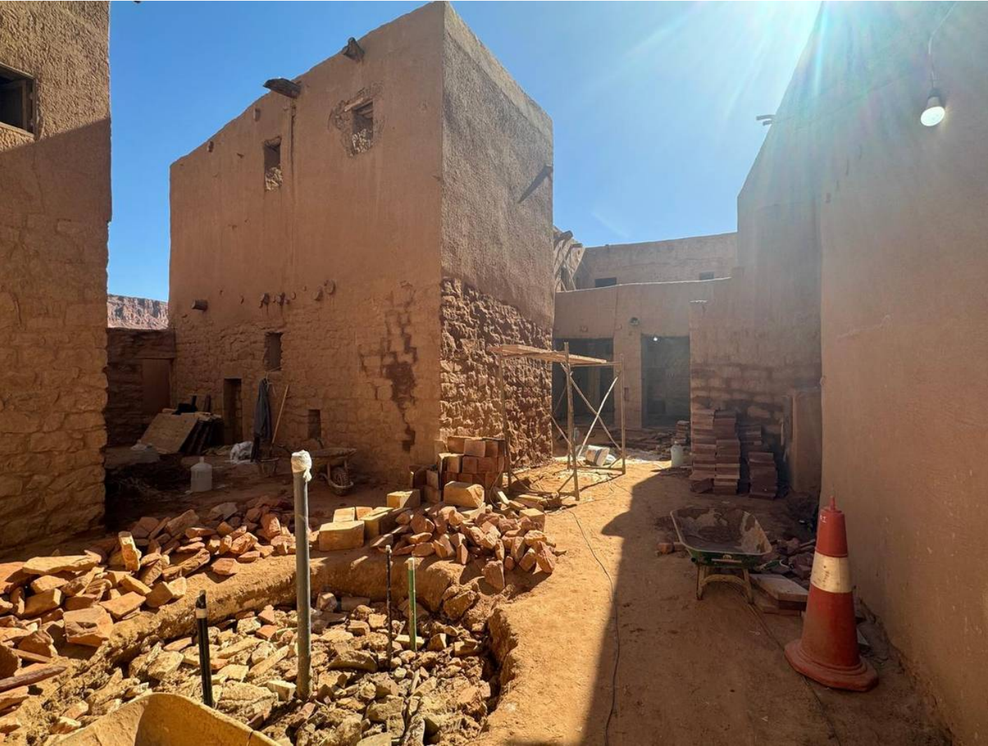
01 Adaptive Reuse Works in Progress
