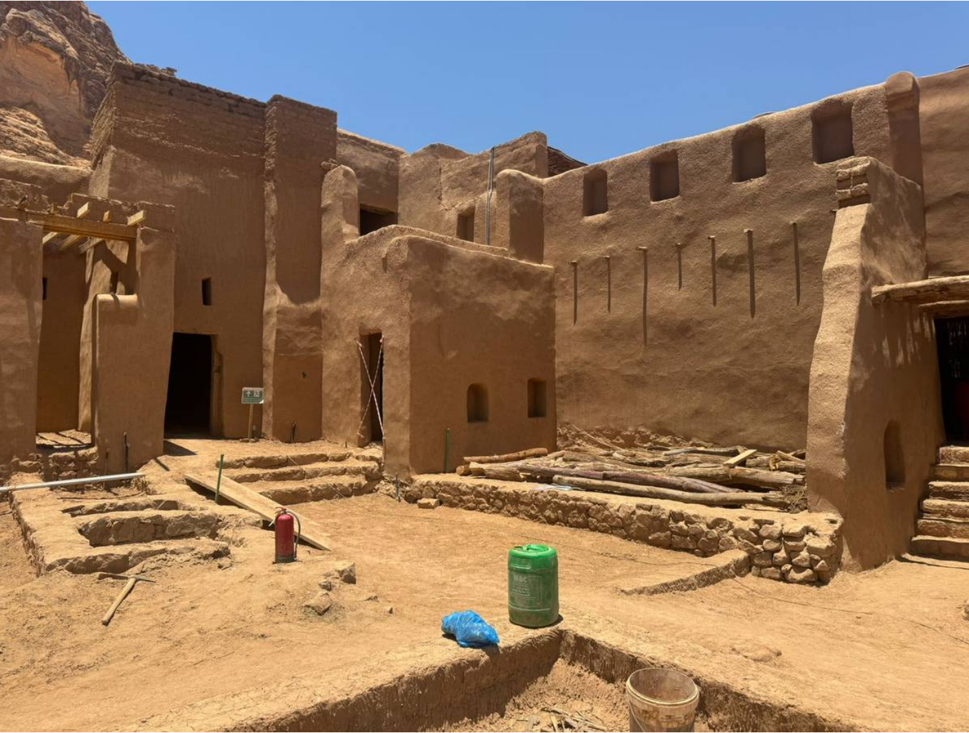
Restoration Works in Progress
