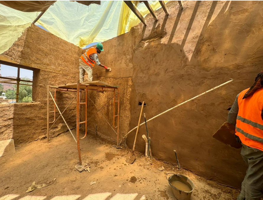
Restoration Works in Progress / View 02
