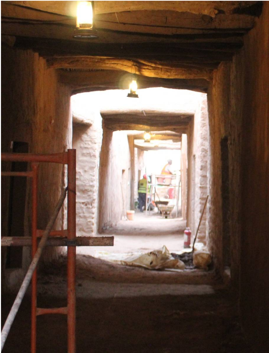
02 Adaptive Reuse Works in Progress
