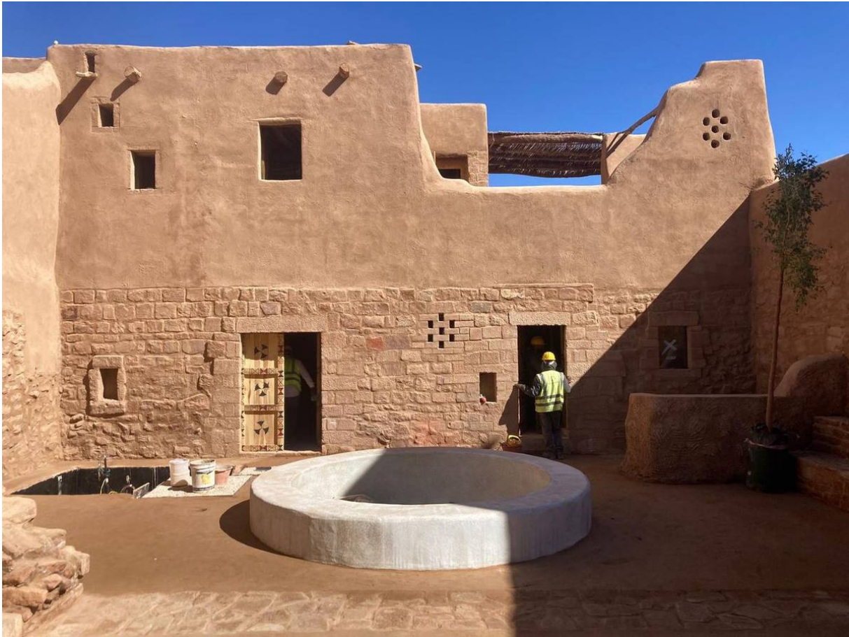
02 Adaptively Reused Condition
