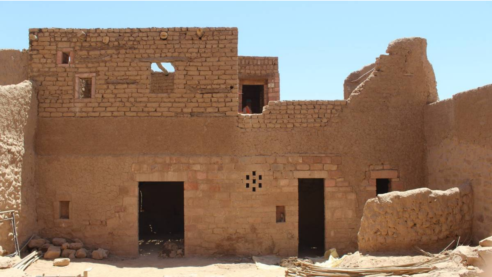
01 Adaptive Reuse Works in Progress
