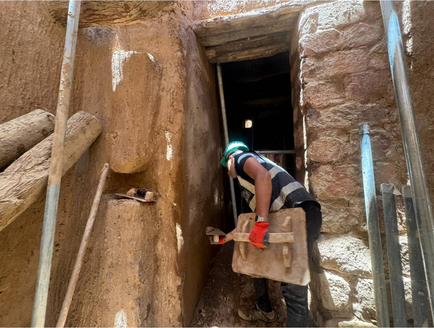
Restoration Works in Progress
