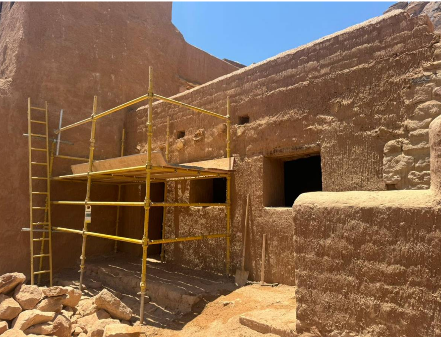
Restoration Works in Progress
