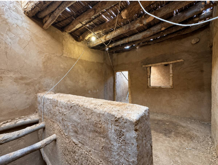
03 Adaptive Reuse Works in Progress
