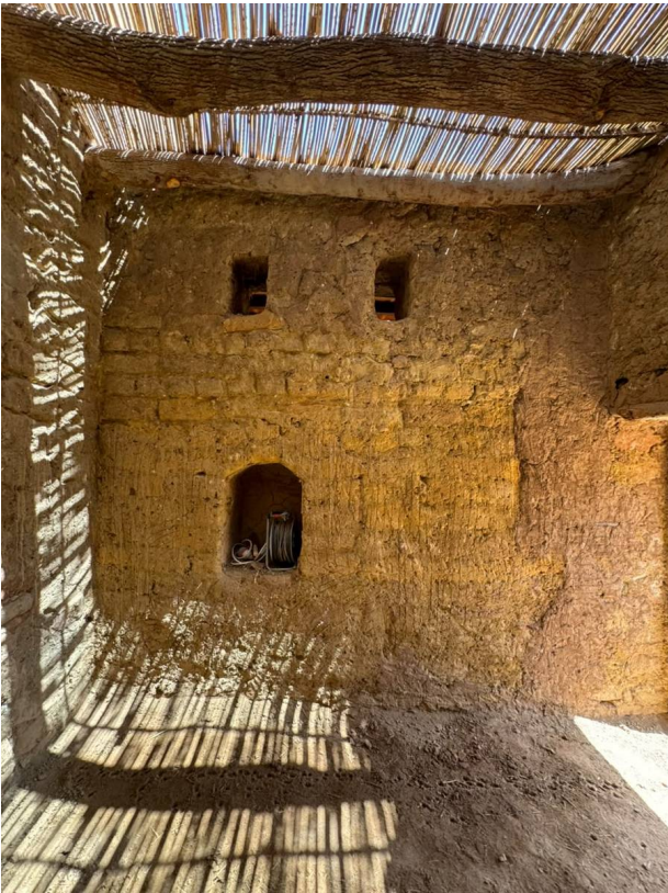
Restoration Works in Progress / View 02
