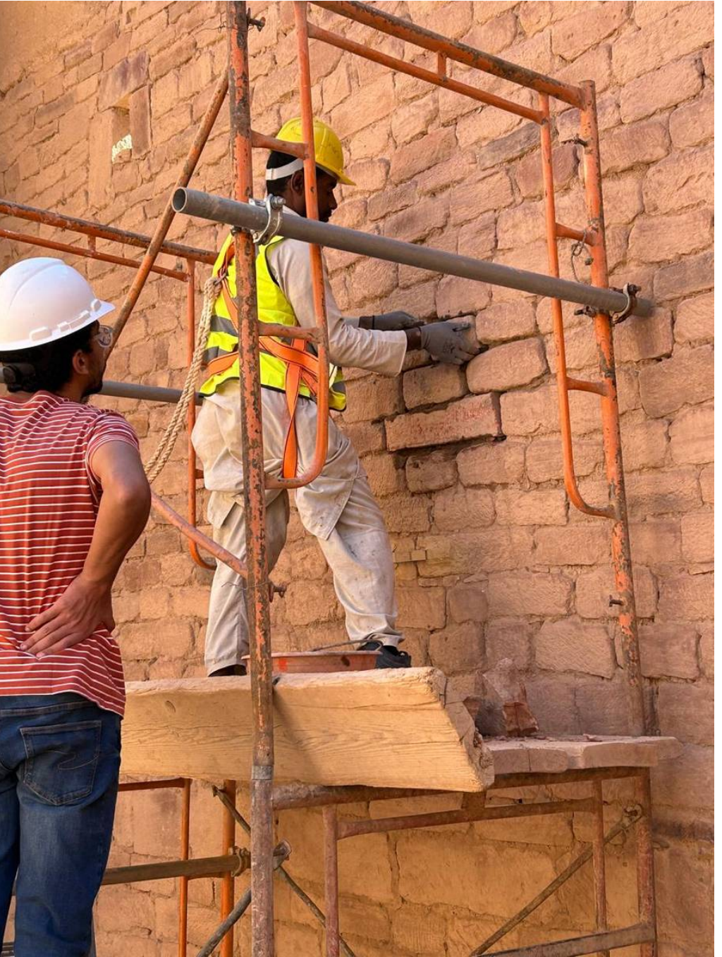
Reassembling and repositioning stones across the crack
