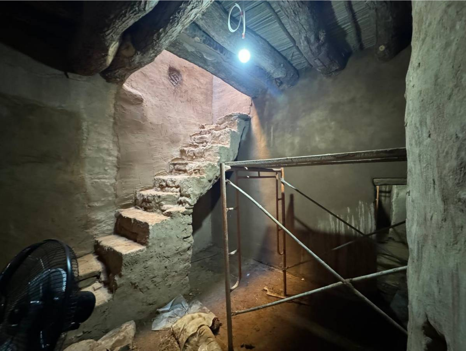
01 Restoration Works in Progress
