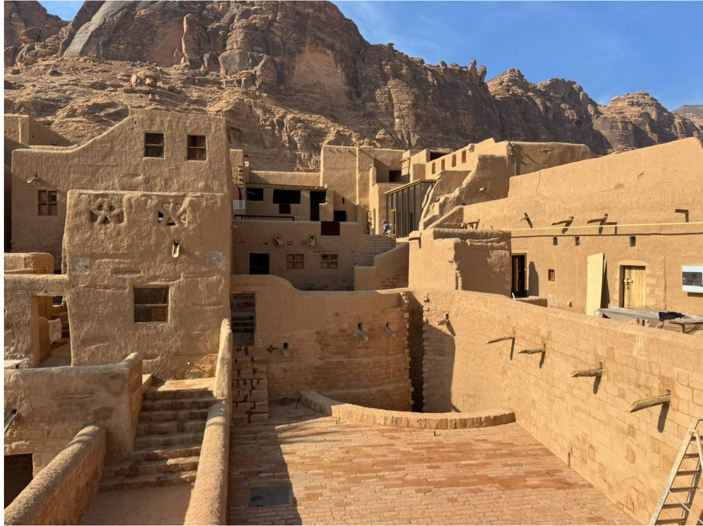
Adaptively Reused Condition
