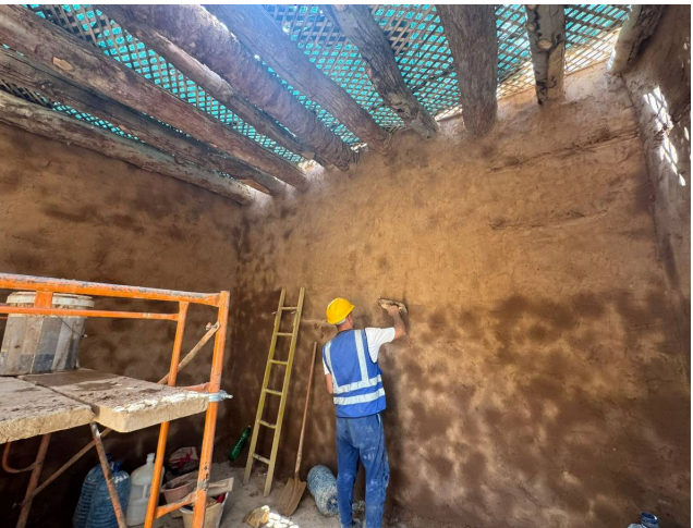
Restoration Works in Progress / View 02
