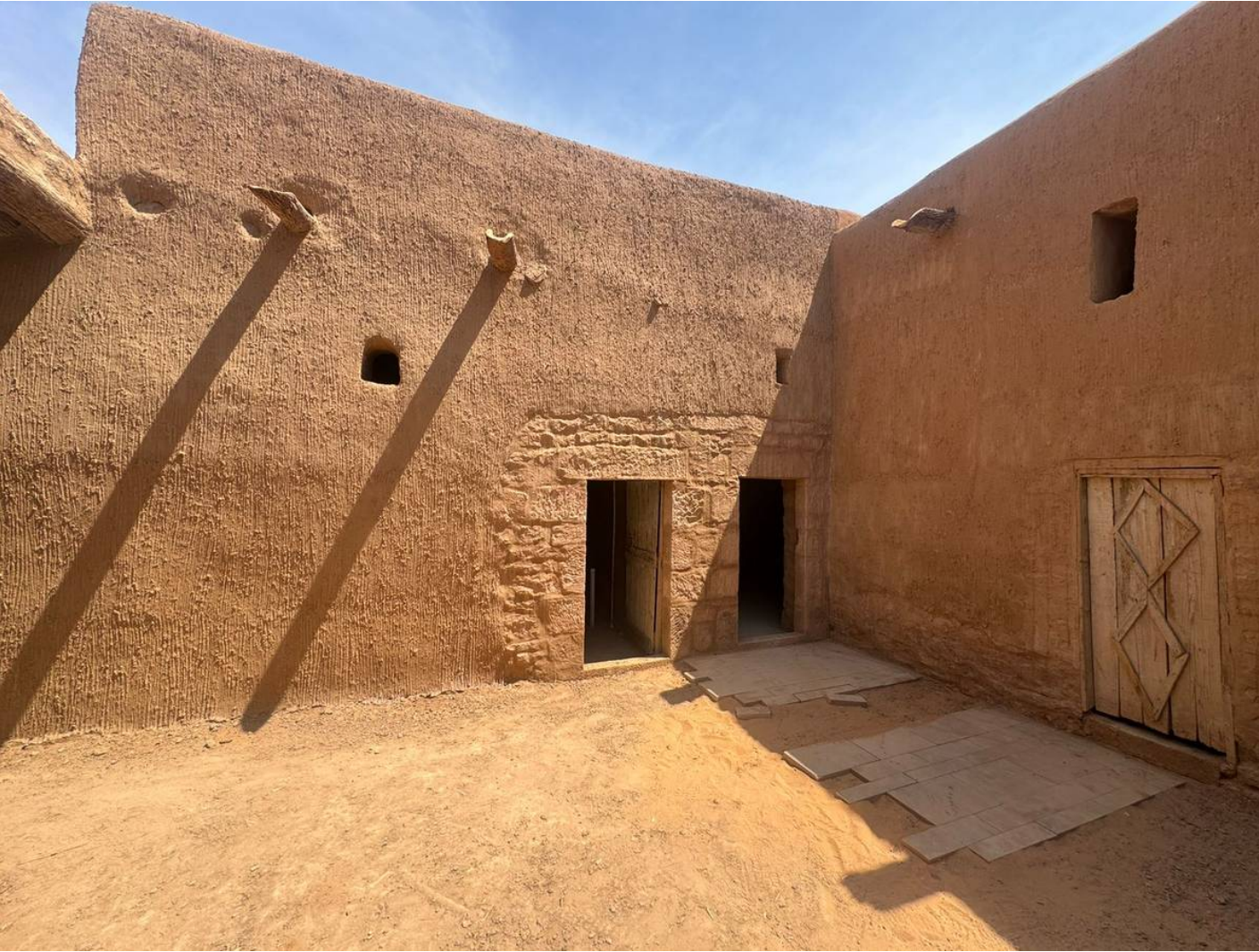
Restored Condition / View 01
