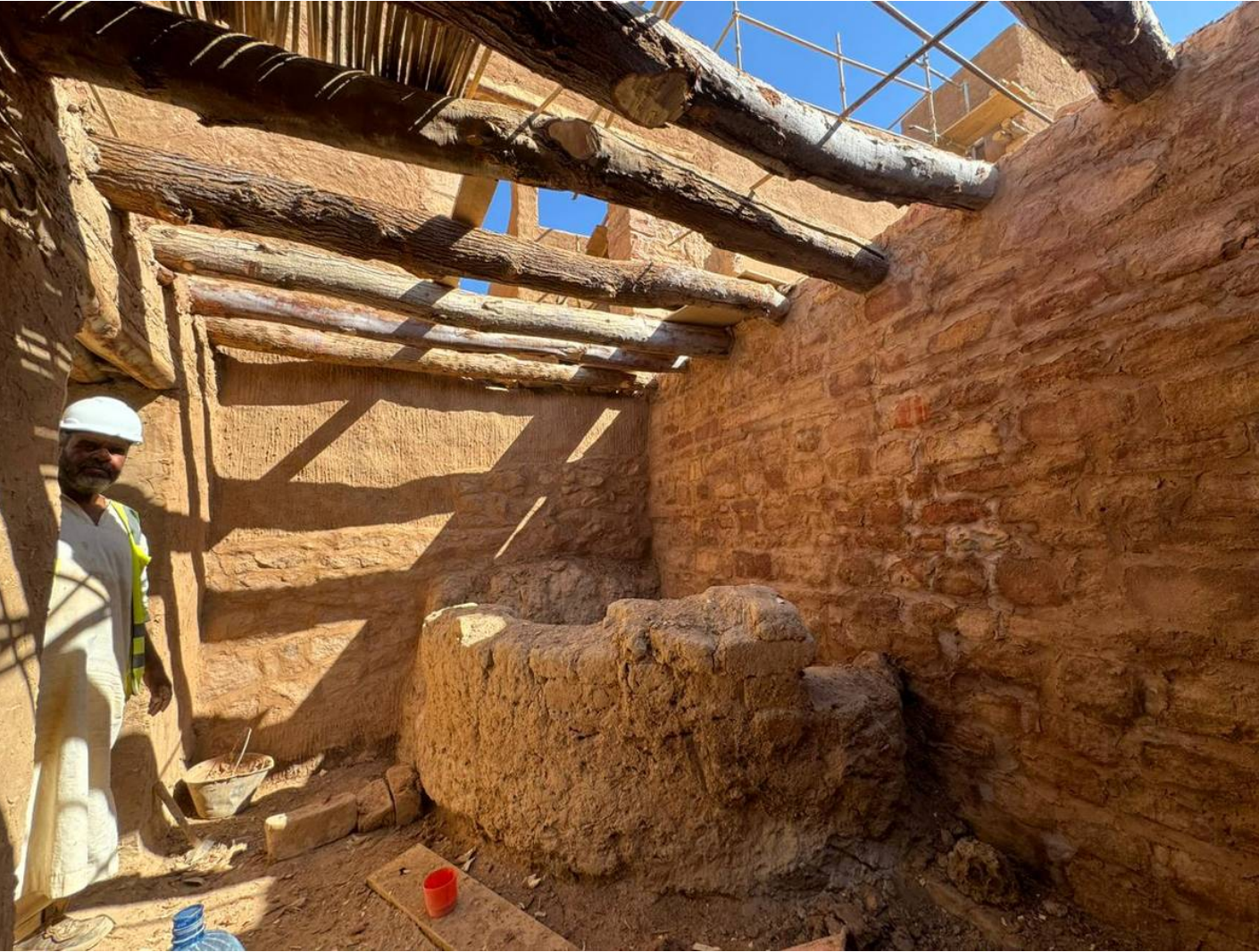
Restoration Works in Progress
