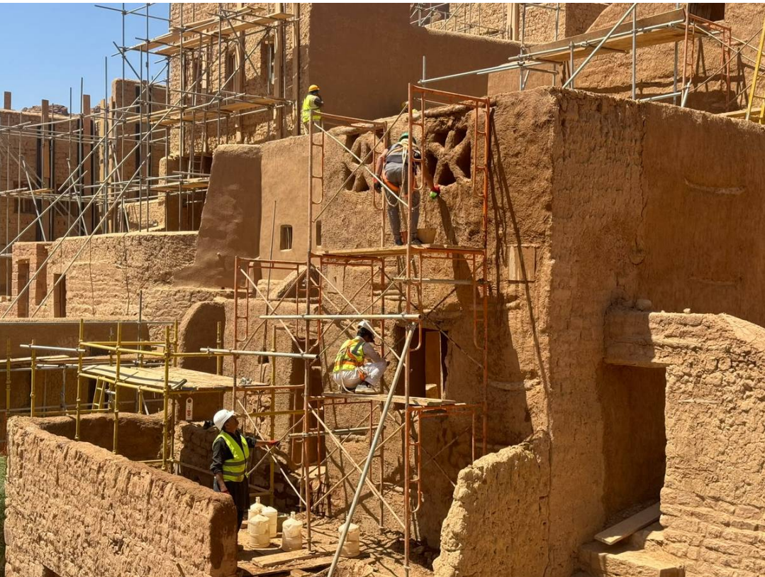
Restoration Works in Progress / View 02
