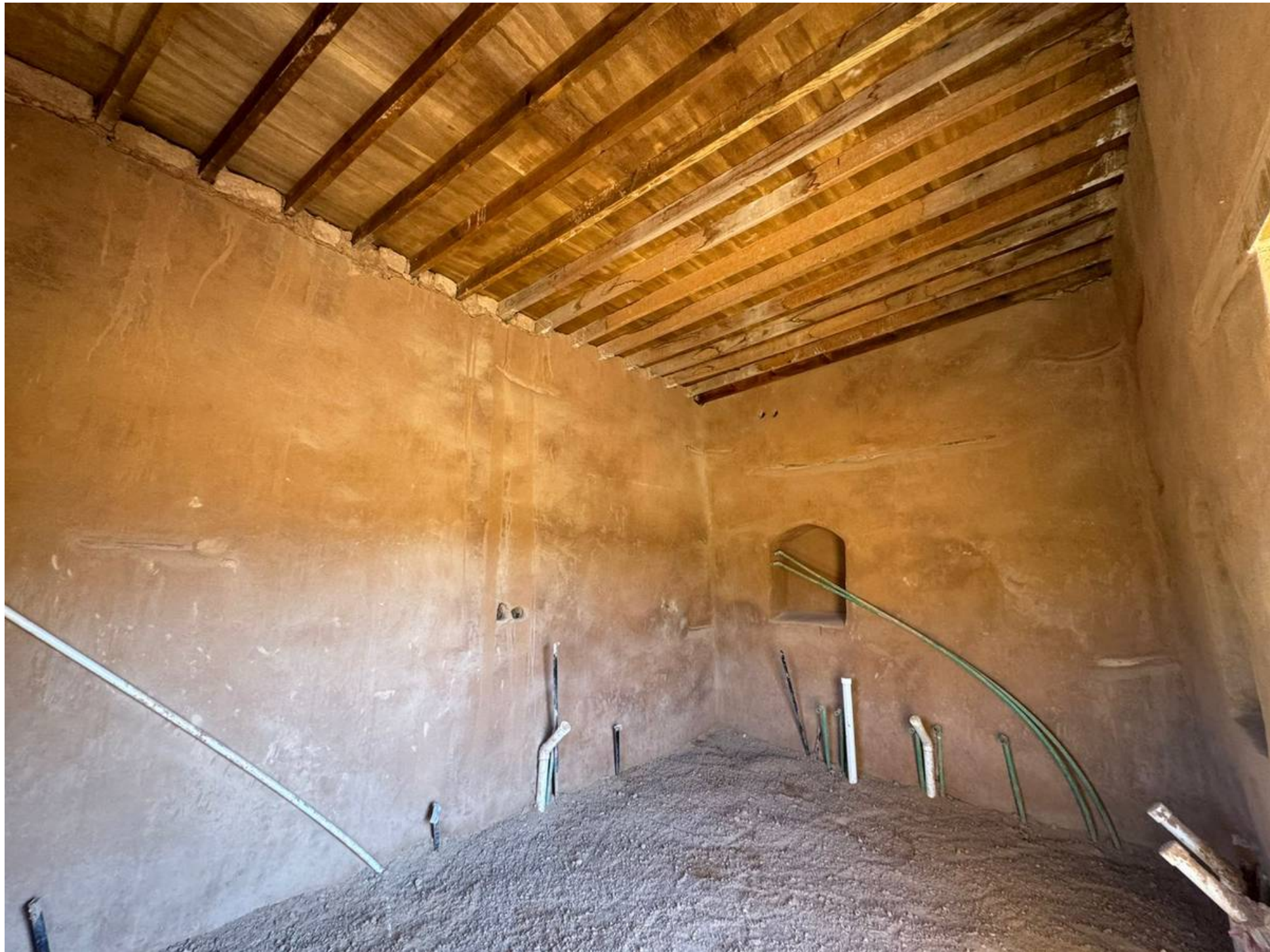
Adaptive Reuse Works in Progress
