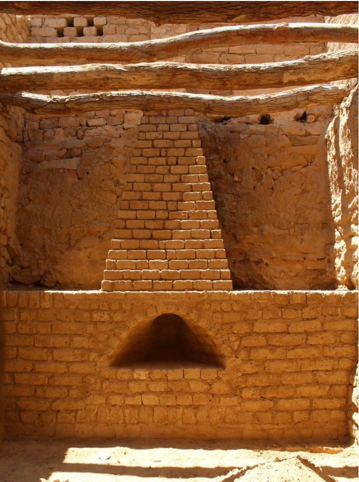
01 Adaptive Reuse Works in Progress
