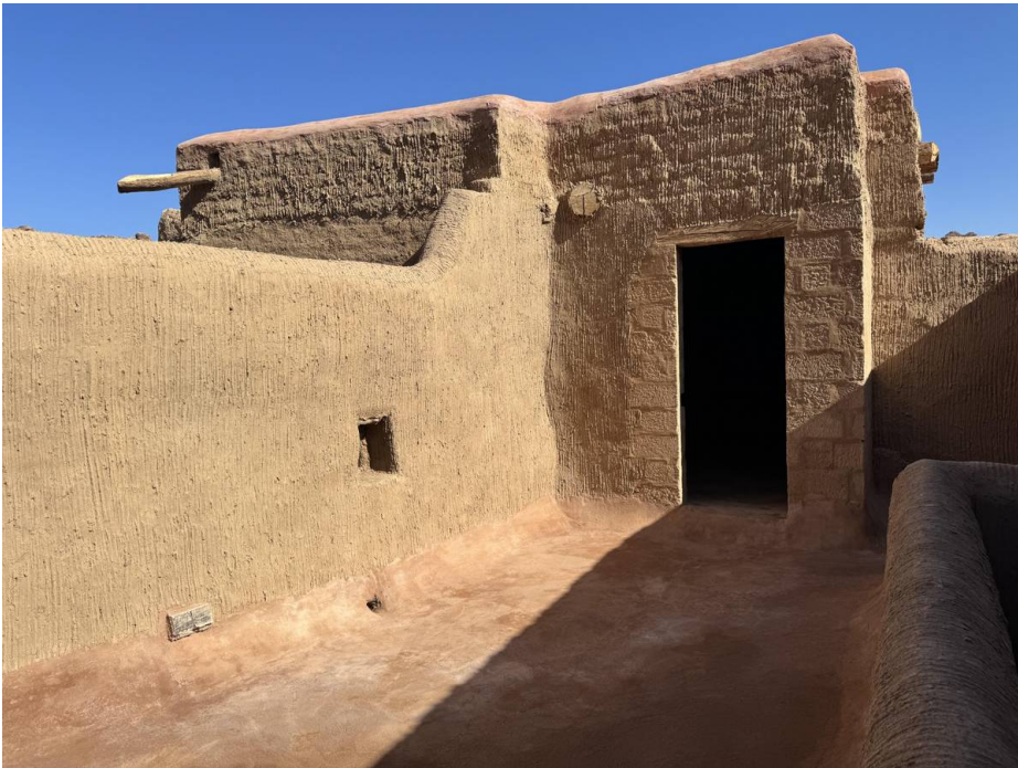
02 D - Restored Condition · First floor
