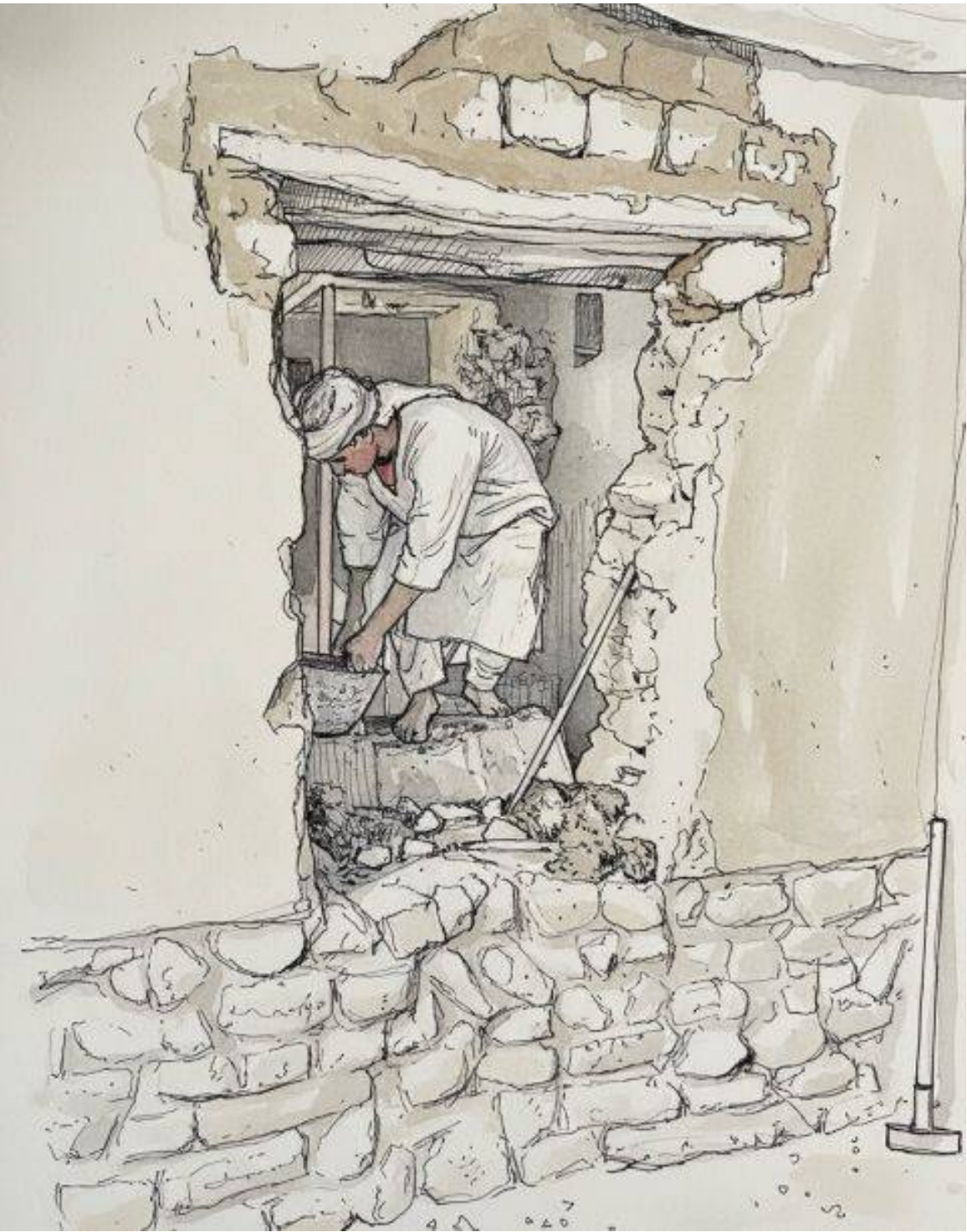
Work at a doorway
