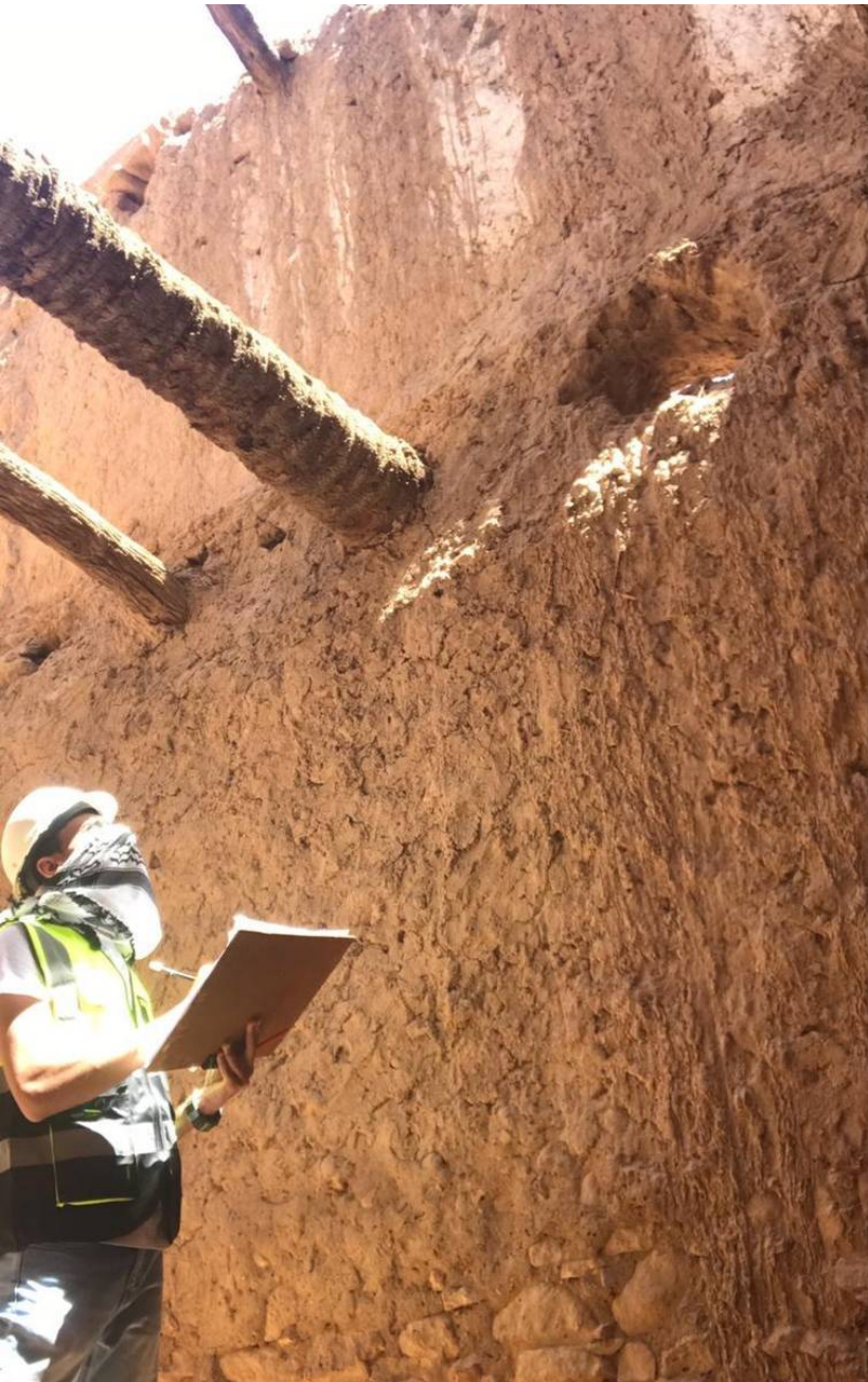
Inspecting earthen walls and timber elements
