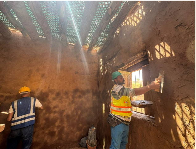
Restoration Works in Progress / View 01
