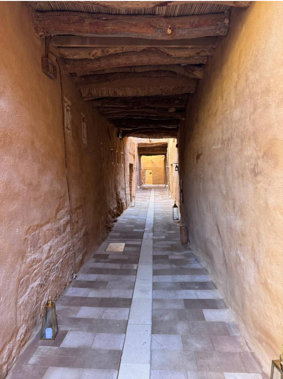
03 Adaptively Reused Condition
