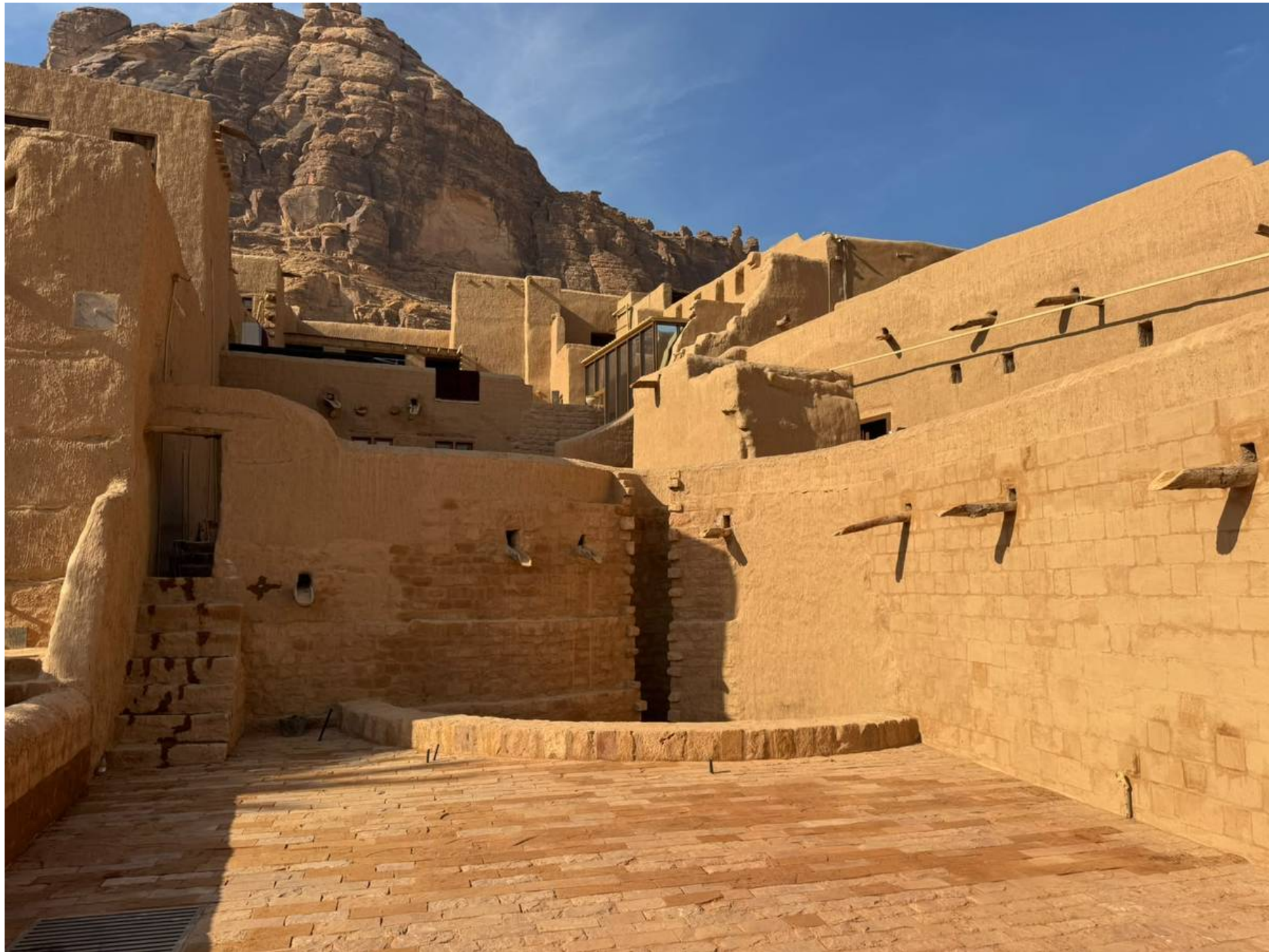
Adaptively Reused Condition
