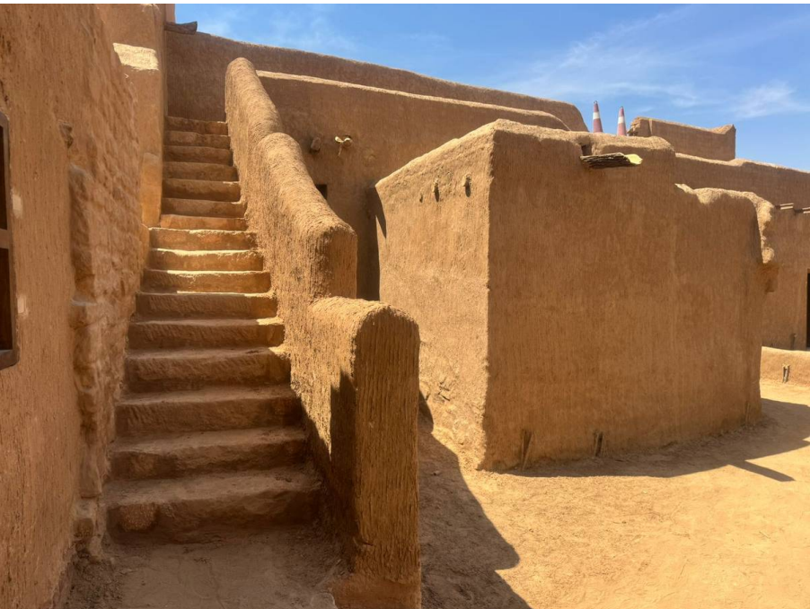
Restored Condition / View 01
