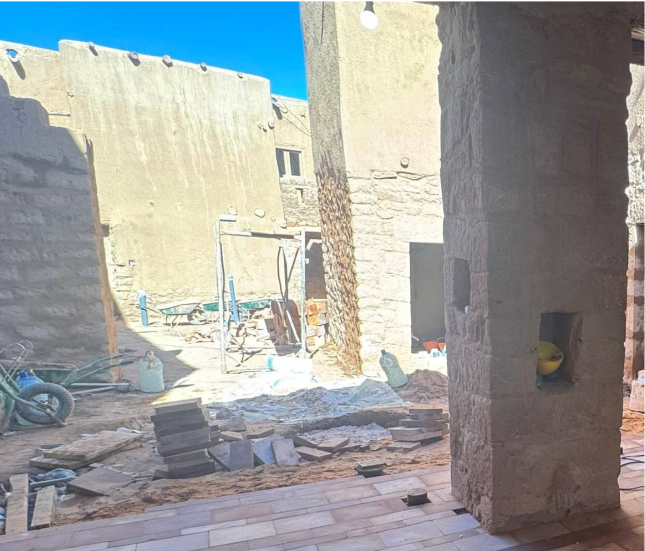
01 Adaptive Reuse Works in Progress
