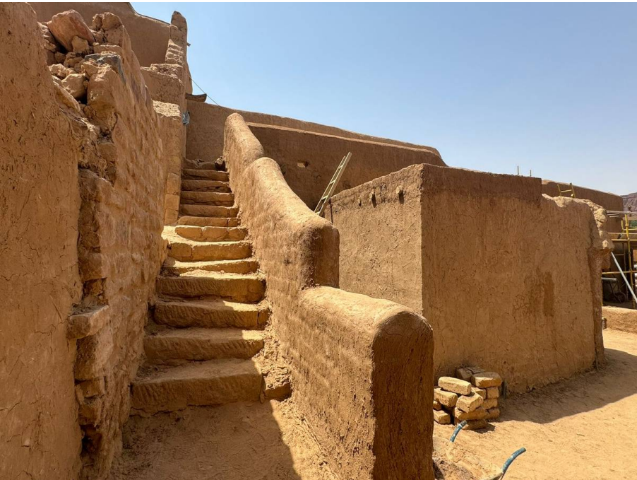
Restoration Works in Progress
