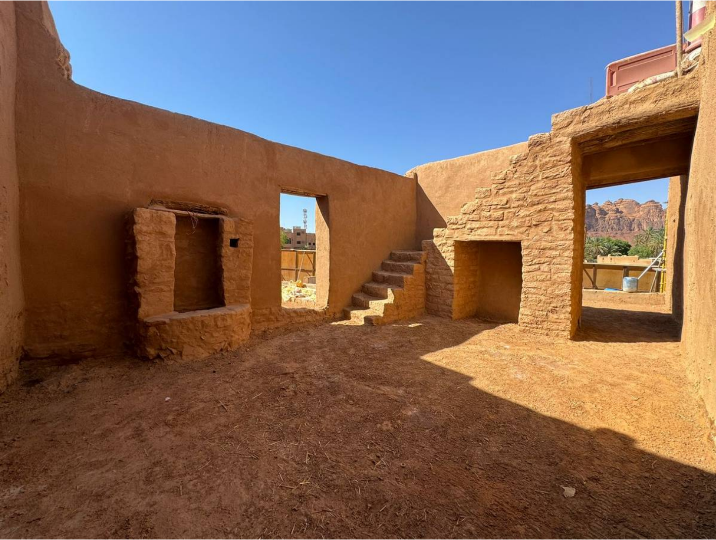
Restored Condition / View 07
