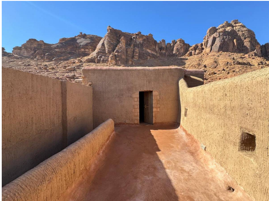
03 E - Restored Condition · First floor
