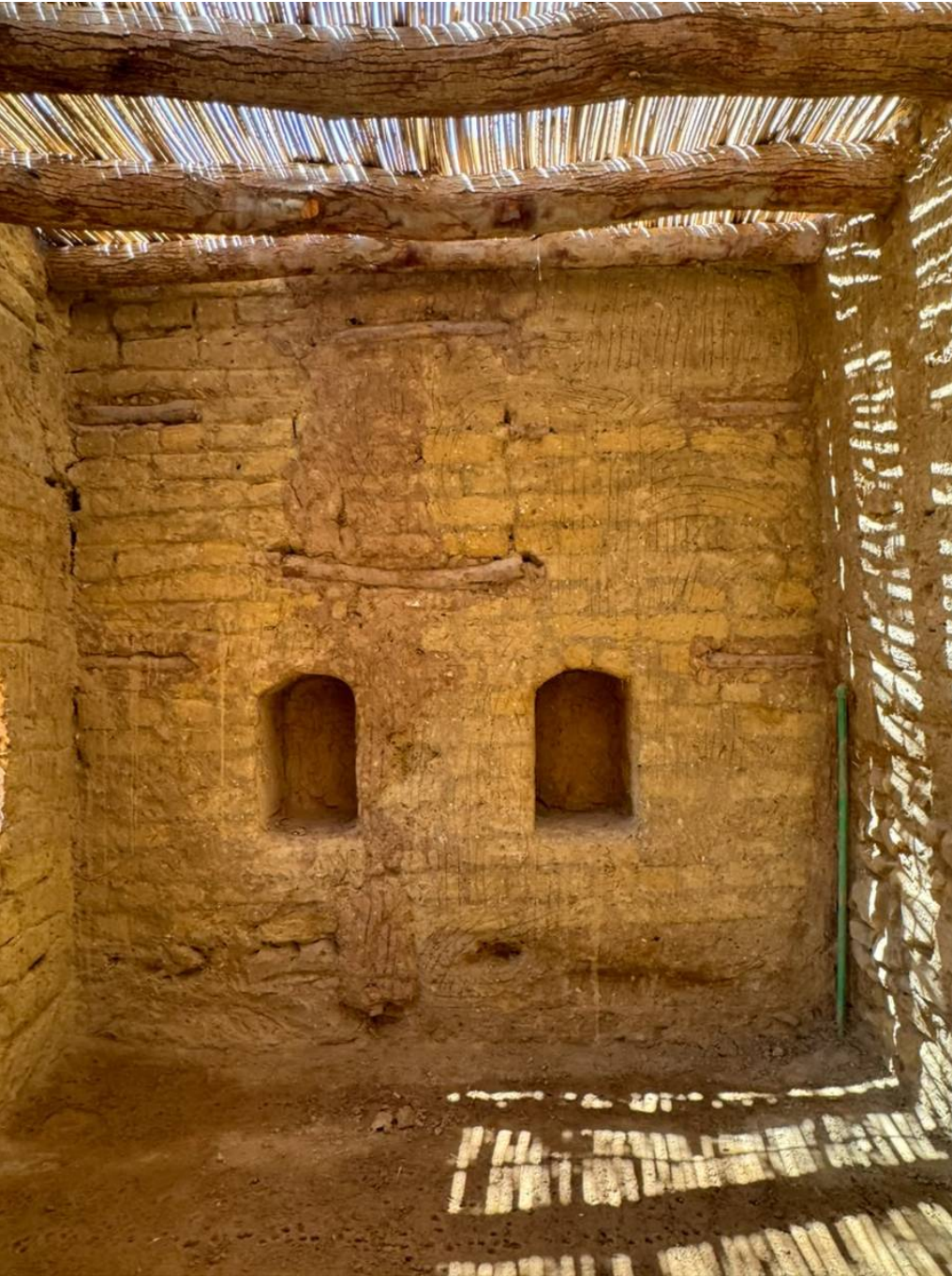
Restoration Works in Progress
