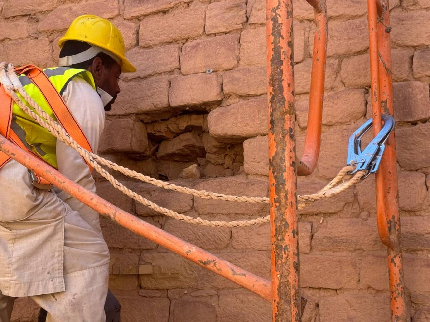
Opened repair area within the stone masonry
