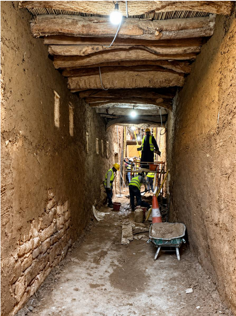
02 Adaptive Reuse Works in Progress
