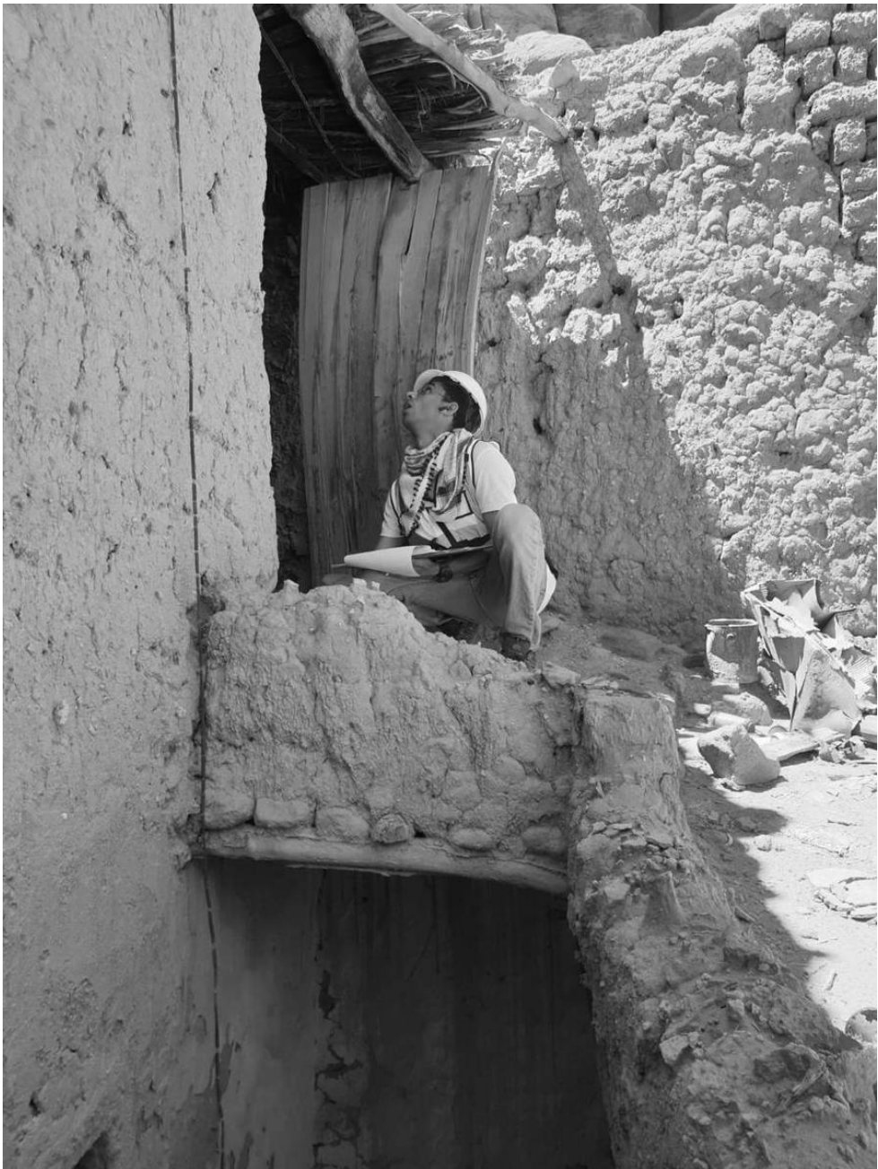
Examining the existing building fabric
