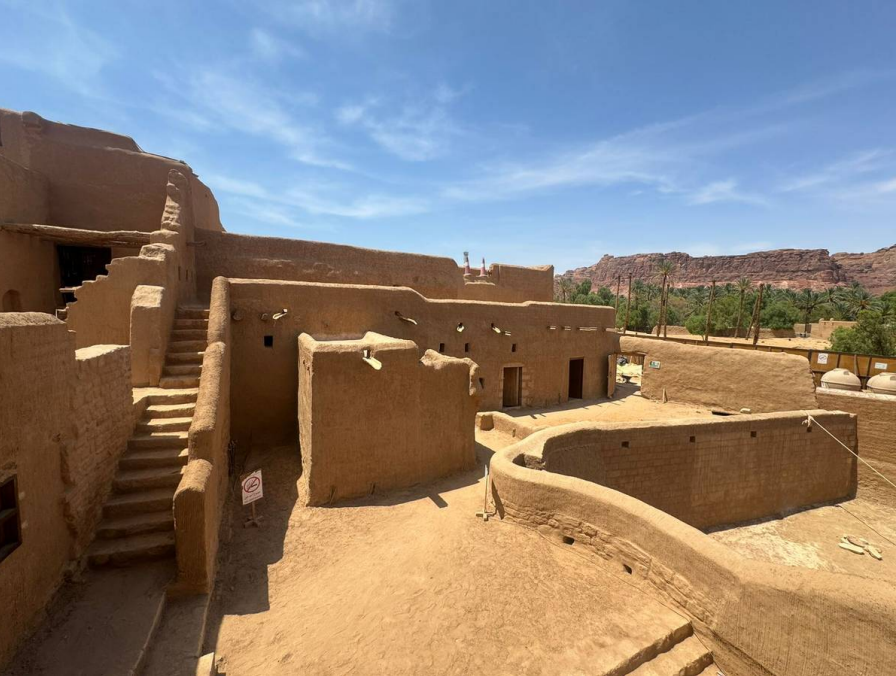
Restored Condition / View 02
