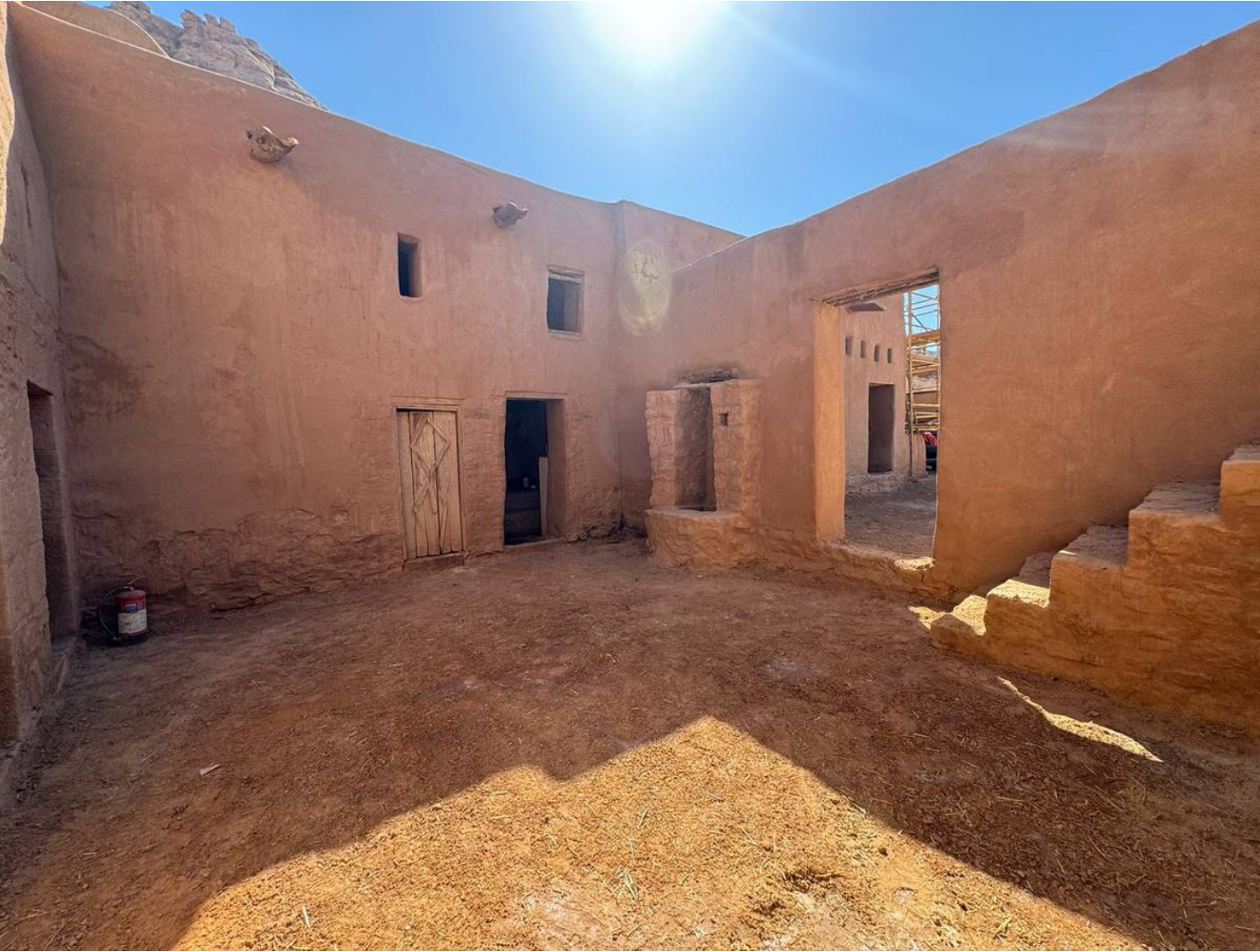
Restored Condition / View 06
