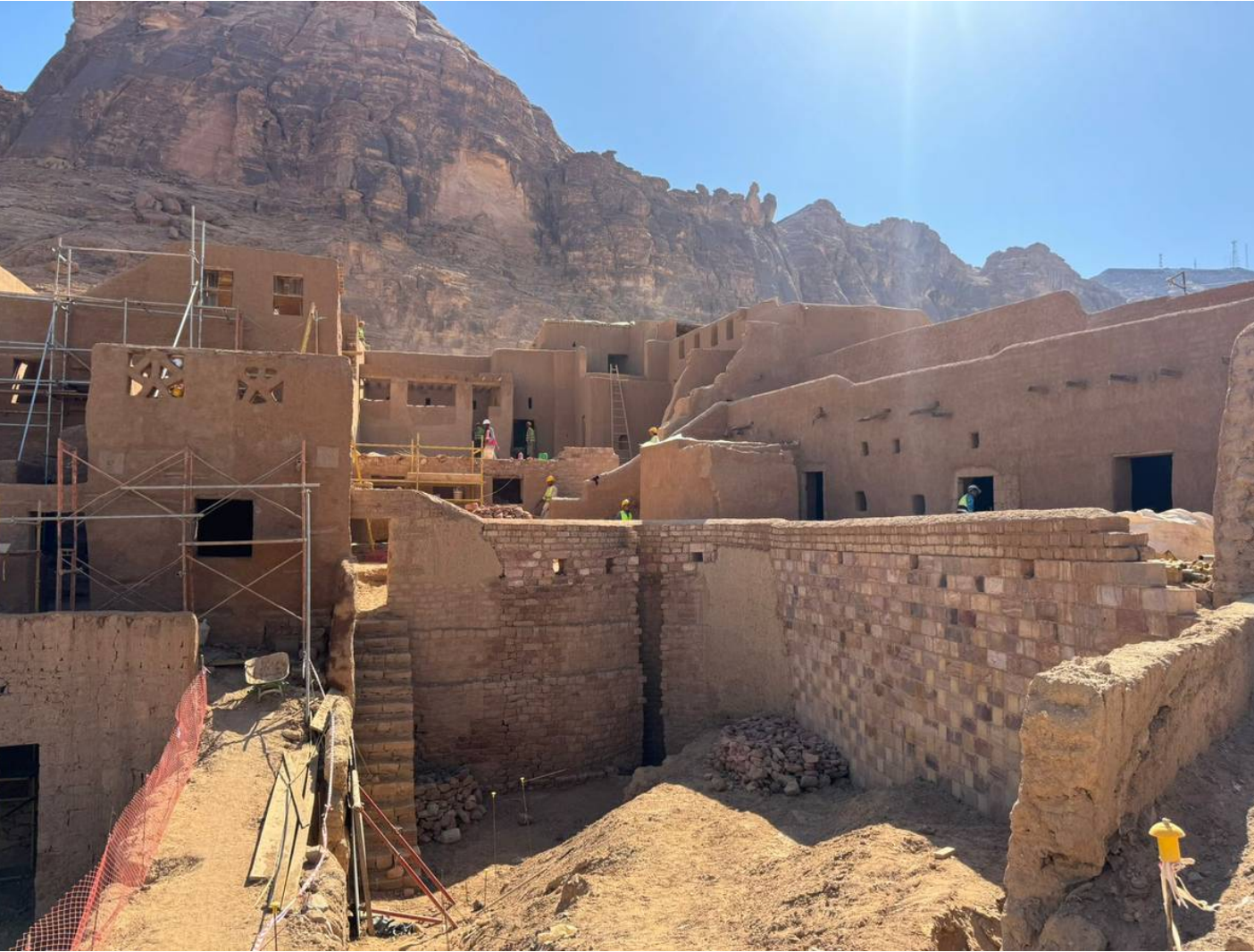
Restoration Works in Progress
