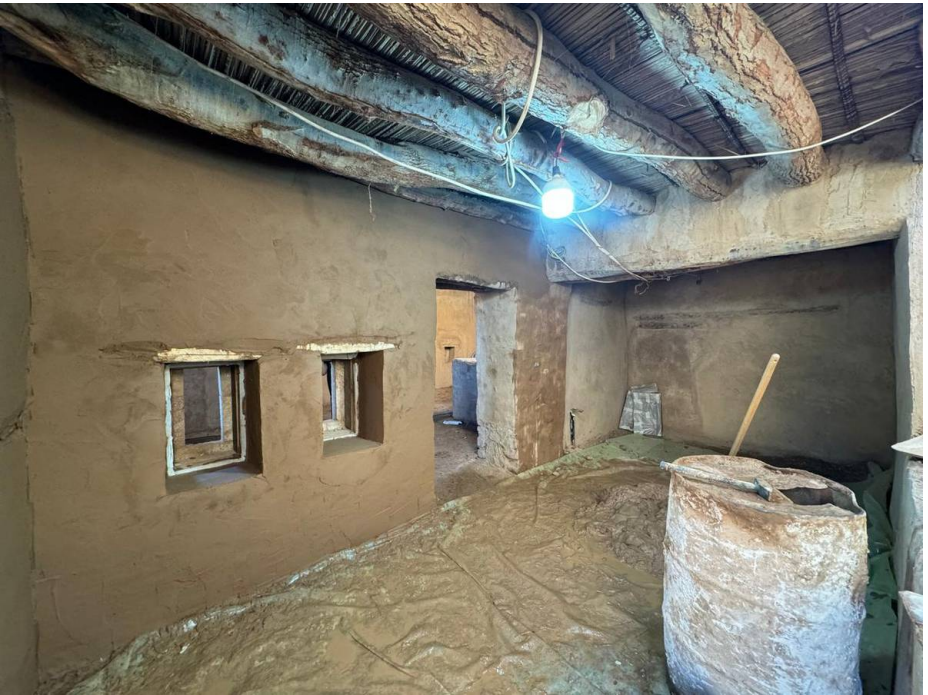
02 Adaptive Reuse Works in Progress
