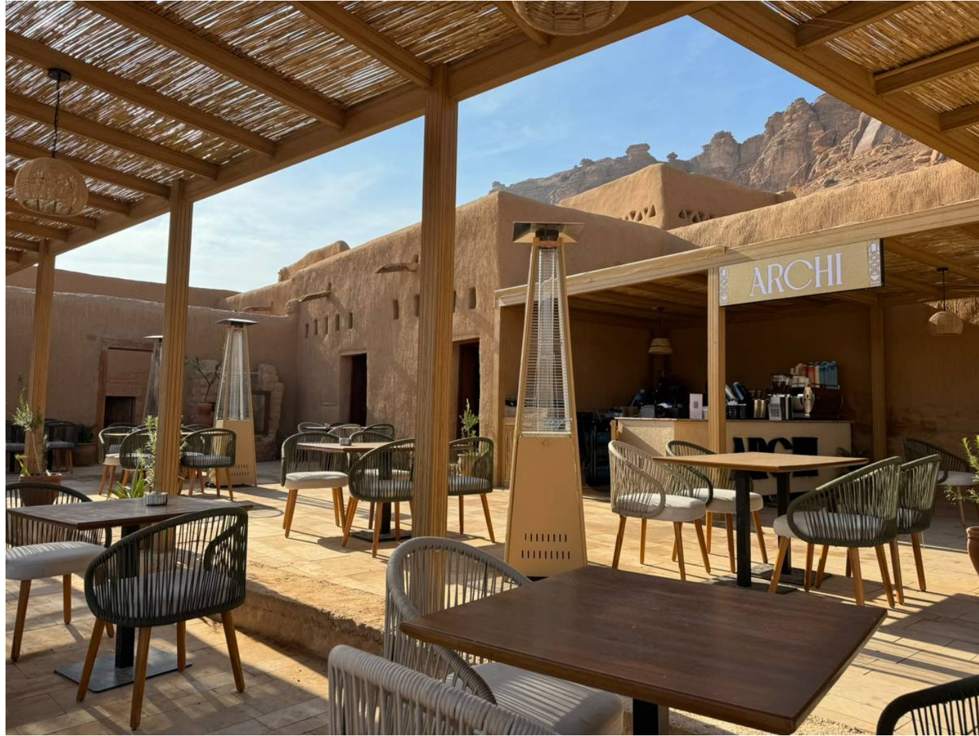
Adaptively Reused Condition
