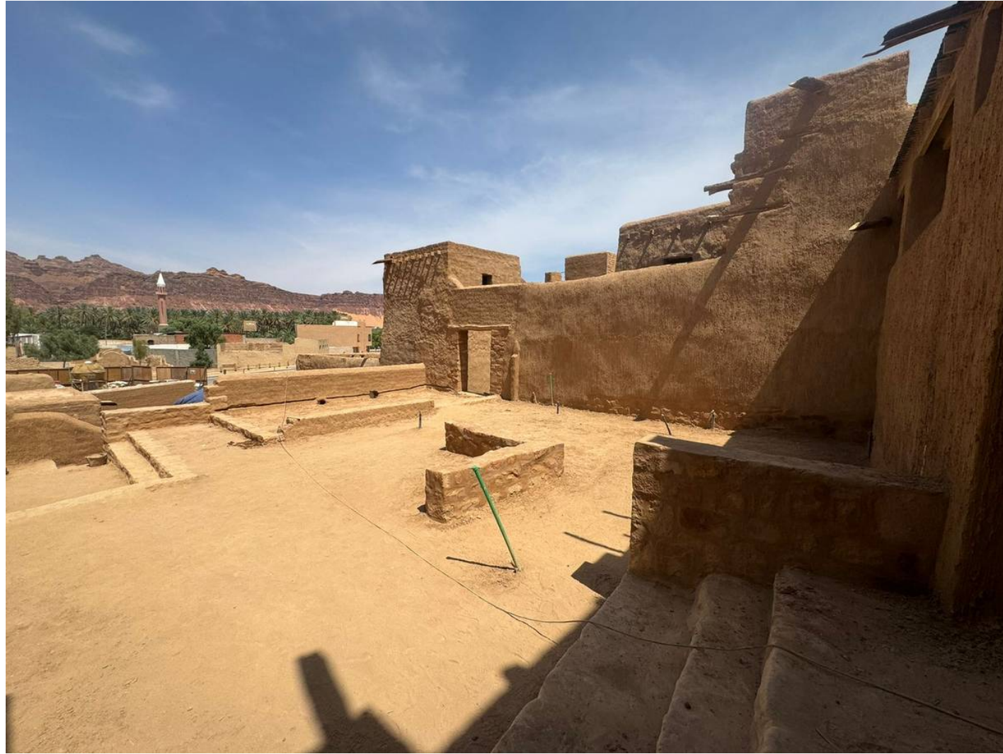
Restored Condition / View 05
