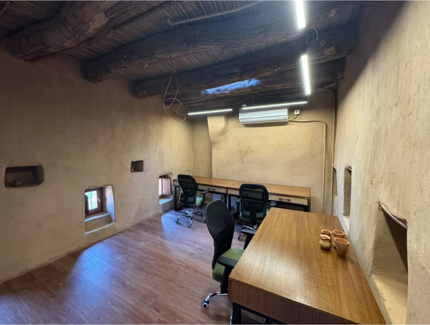
Adaptively Reused Condition
