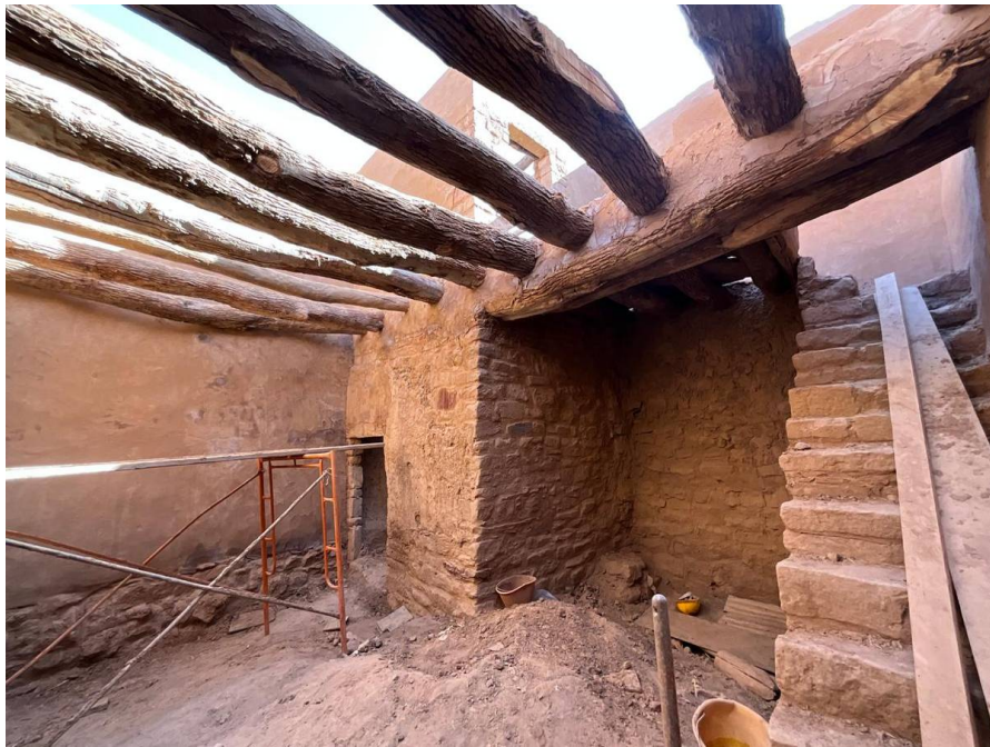
02 Restoration Works in Progress
