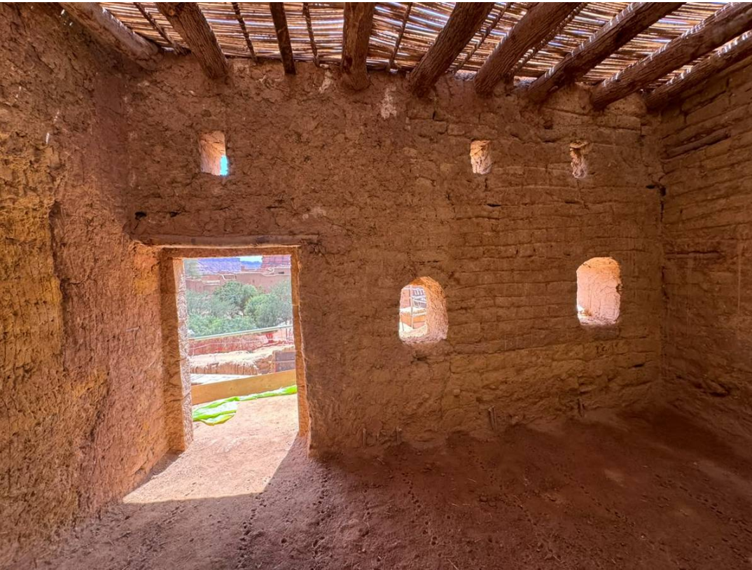
Restoration Works in Progress / View 01
