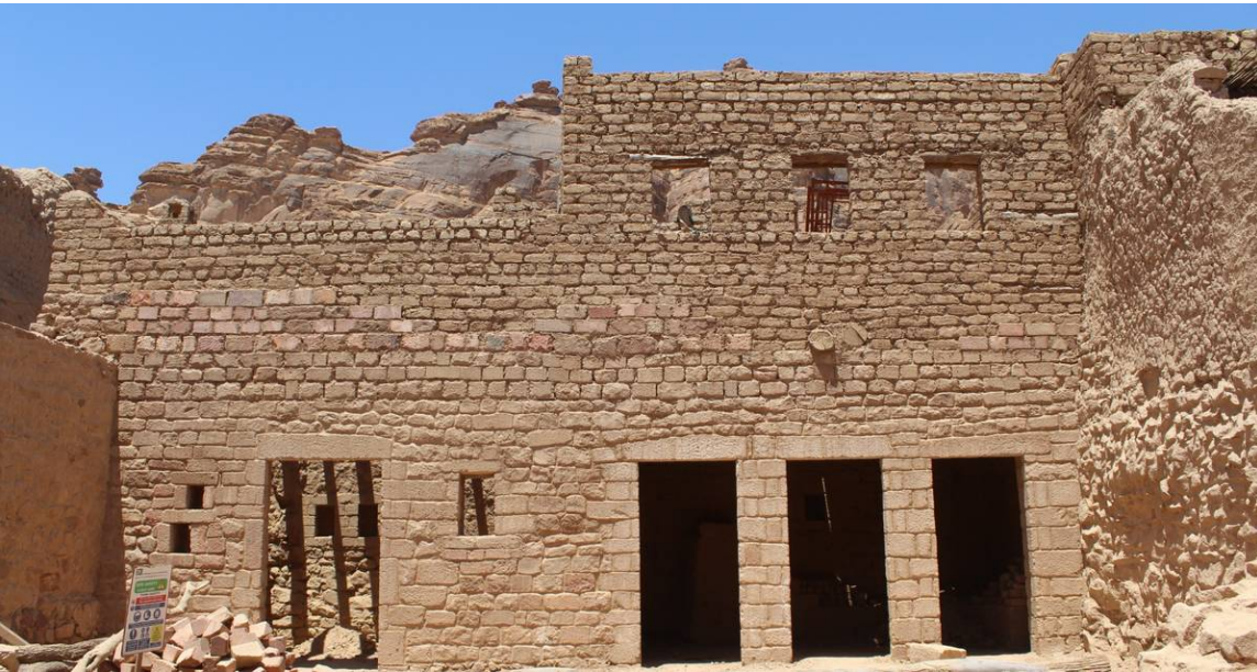
01 Adaptive Reuse Works in Progress
